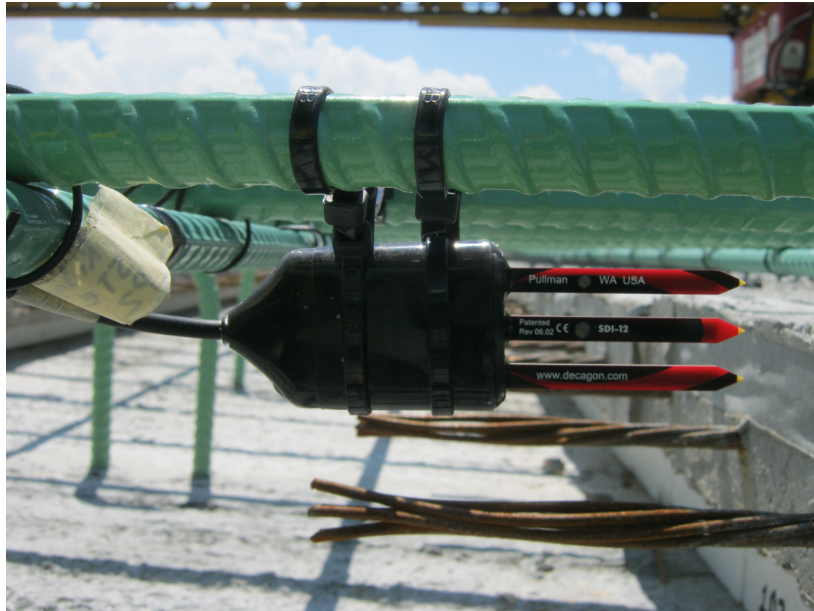
Figure 3-2: Sensor installed just below the top mat of reinforcement.
