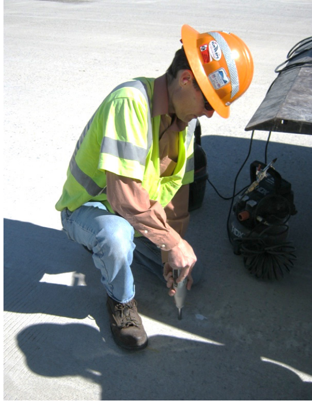
Figure 3-12: Schmidt rebound hammer testing.
