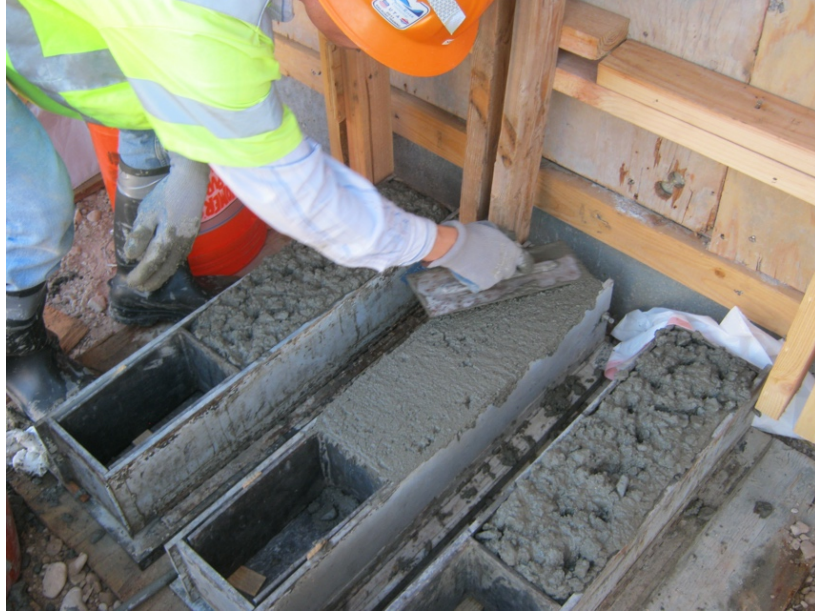
Figure 3-6: Casting of beam specimens during construction of bridge decks.
