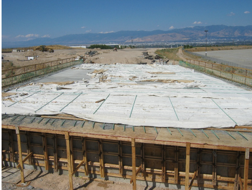
Figure 3-4: Covered bridge deck during curing.
