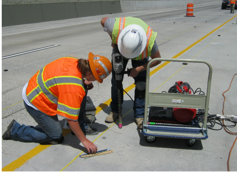
Figure 3-13: Concrete sampling for chloride concentration testing.
