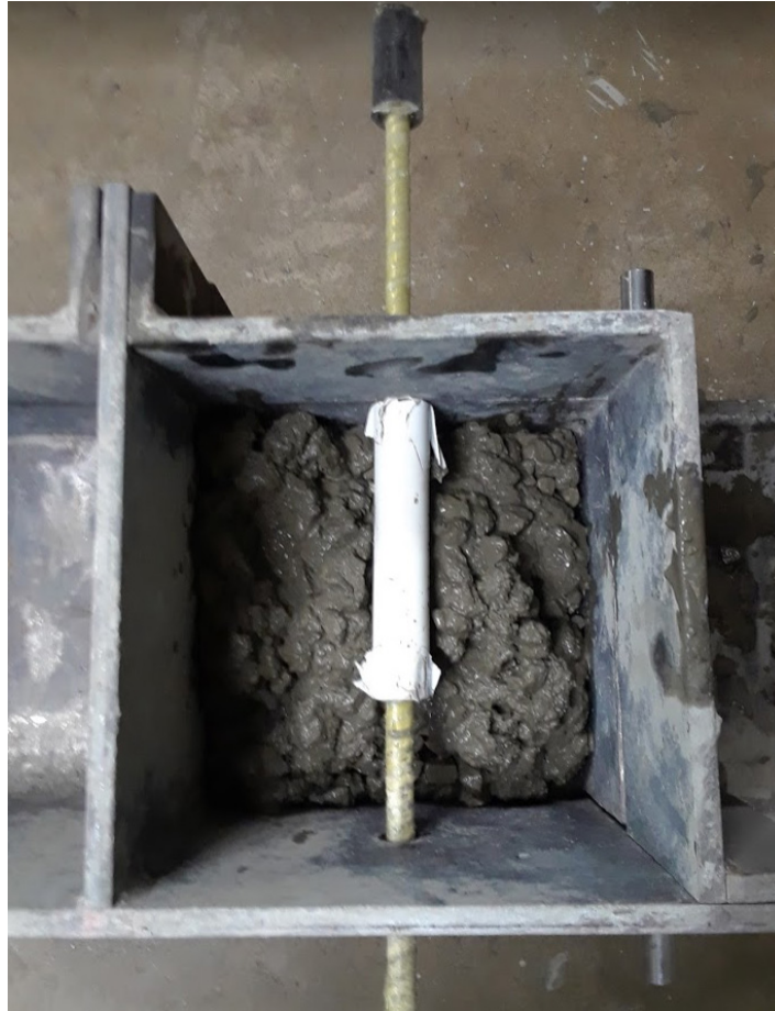
Figure 3-14: Rebar Positioning and PVC in Form
