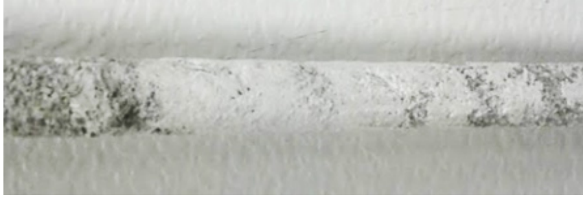
Figure 4-40: Concrete Shear Failure on American Fiberglass Sand-coated Rebar
