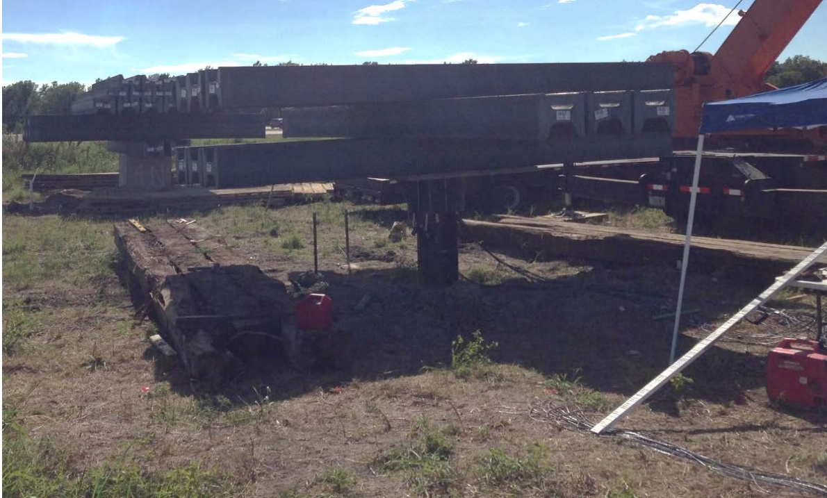
Figure 4.4-8 Photo of the loading configuration completed.
