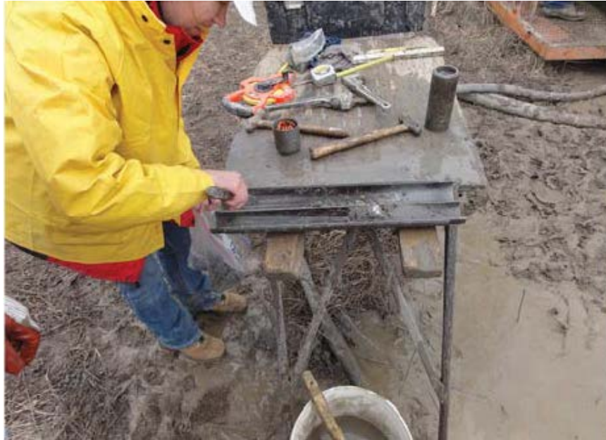
Figure 3.1-2 Photo of a student working with a split spoon sampler during SPT testing at TATS field site (Bey 2014).
