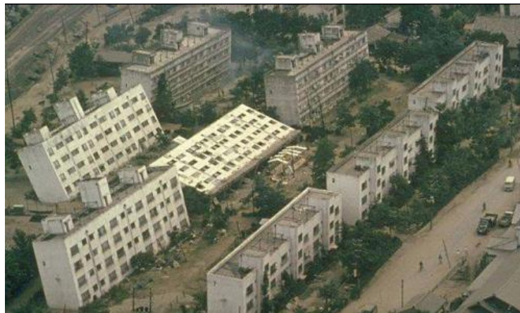
Figure 3-21: Apartment buildings after the 1964 Niigata, Japan earthquake.
