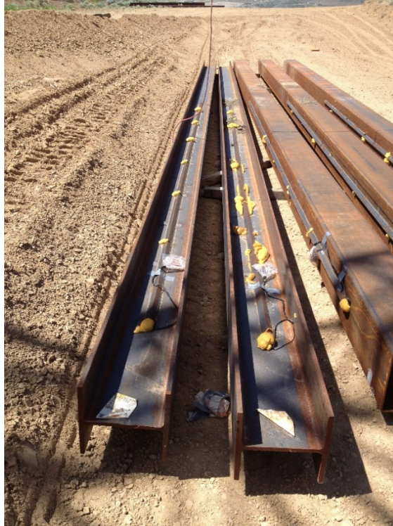
Figure 4-4: Strain Gauges Encased in a Steel Angle
