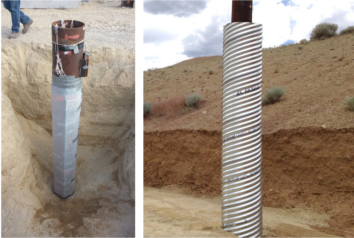
Figure 3-3: (Left) Round Pile with HDPE, (Right) Round Pile with CMS
