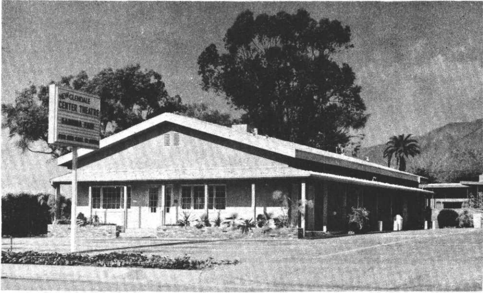
Doran Street Theatre Exterior
