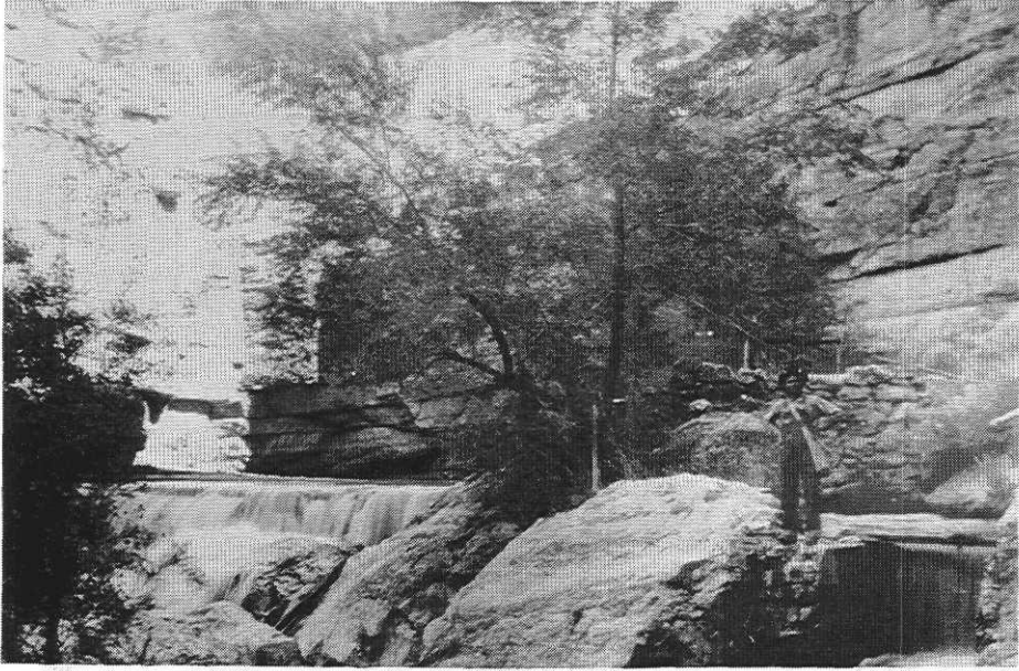
Figure 19. Dam and control gate. William Hinton pictured (courtesy Fern Reeve).
