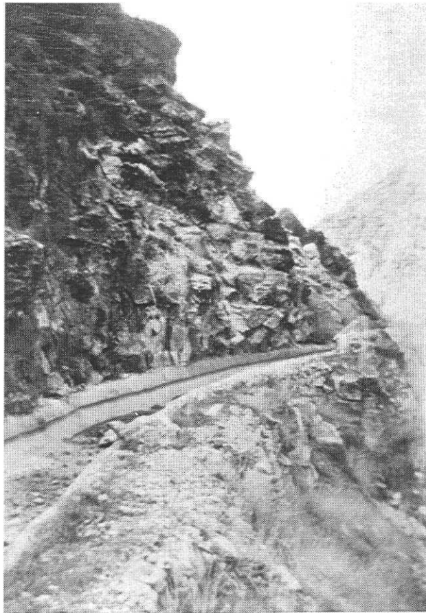
Figure 23. Concrete portion of canal (Lynn Clark Southern Utah Historical Collection donated by Wazel and Keith Hall).
