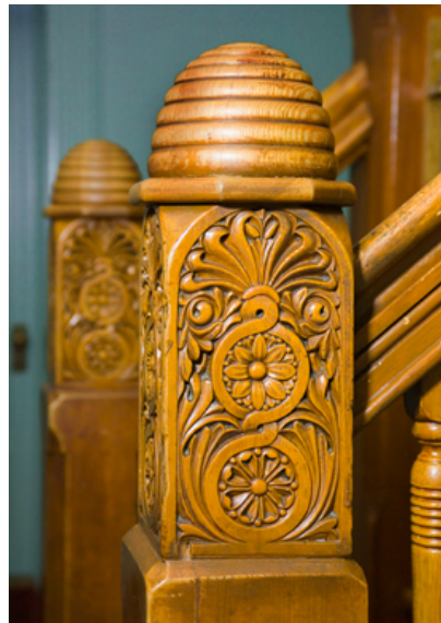
Posts and stair rails at Brigham Young's Beehive House in Salt Lake City.
