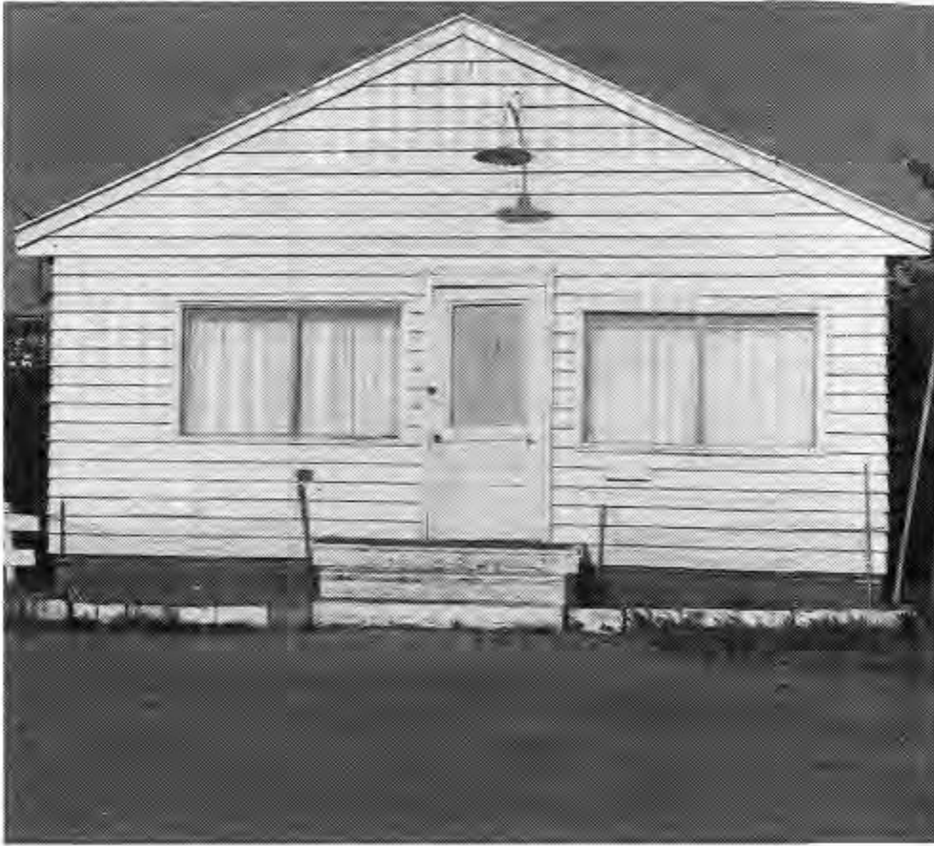
FIG. 5. This converted gasoline station was purchased for the Native branch near the Cote Reserve in eastern Saskatchewan. Small buildings such as this one are often used when branches are just becoming established. Photographed 1978.
