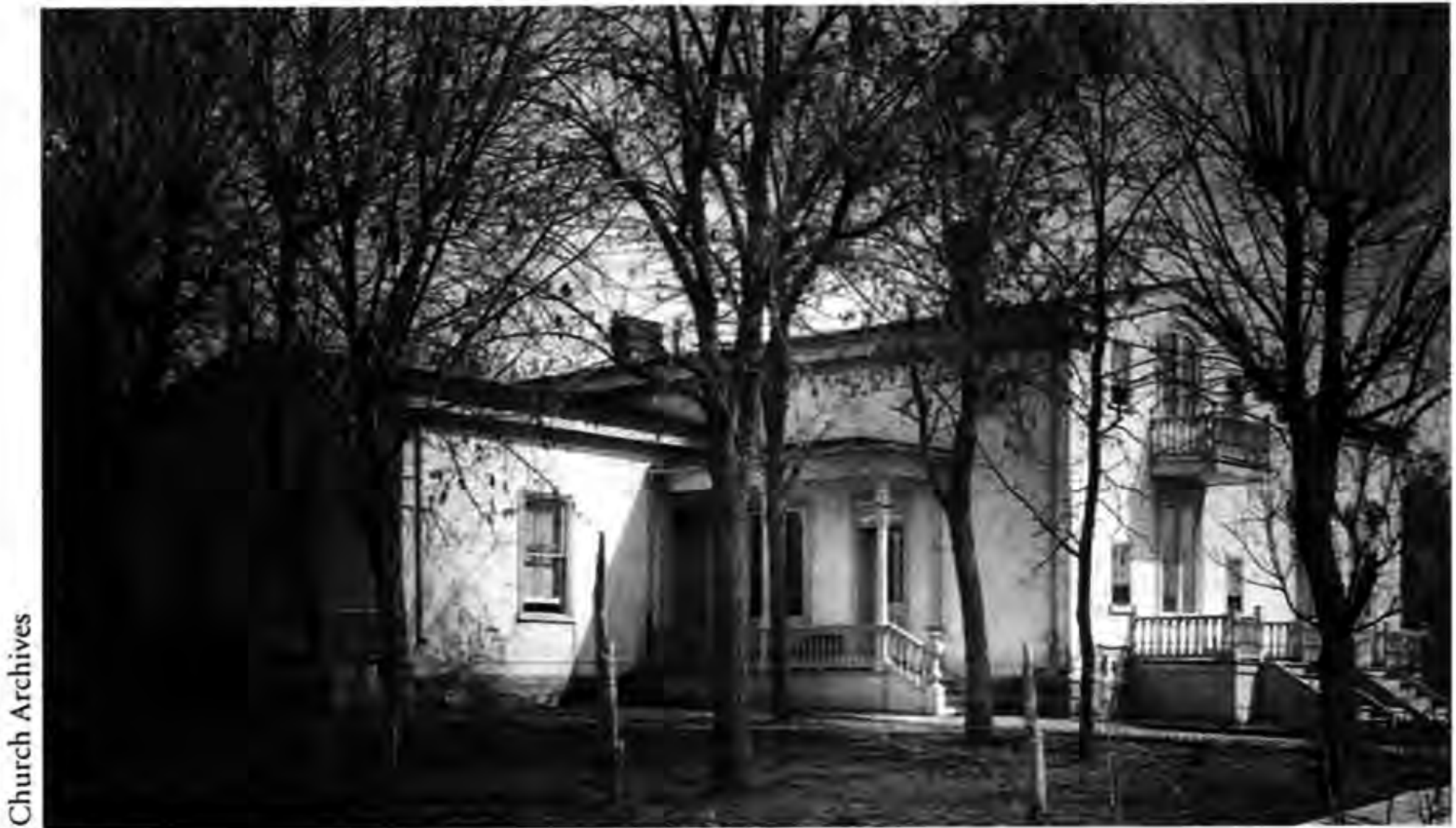
FIG. 3. White House, ca. 1888. Brigham Young erected the White House from 1849 to 1851 as a residence for wife Mary Ann Angell and their five children. Standing on the north side of what is today South Temple between the Eagle Gate and A Street in Salt Lake City, the house was built of adobe bricks and covered with plaster. This photograph by Charles R. Savage shows the outlines of the shingled roof, said to be the first in Utah.
