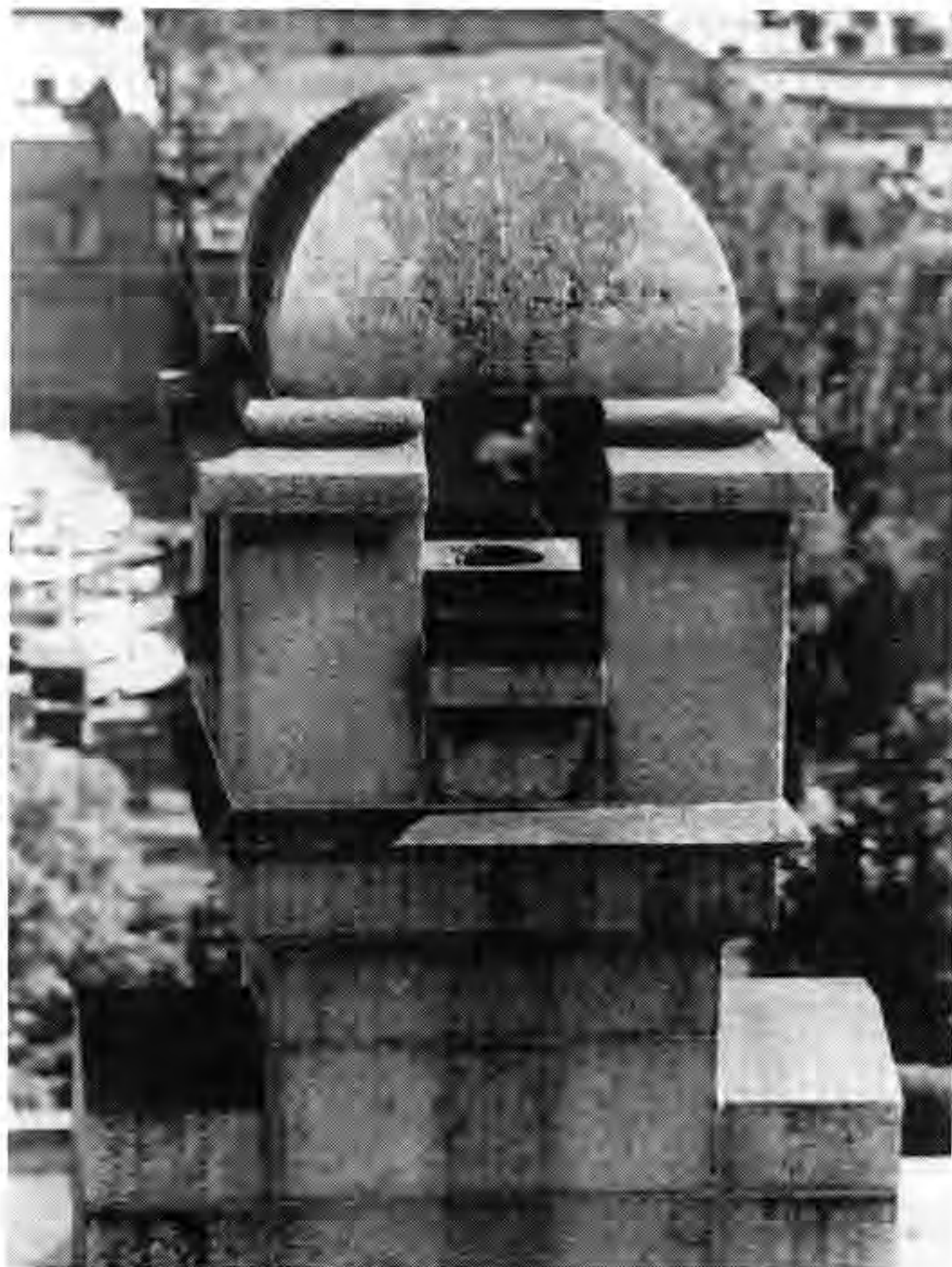
Flued buttress. Note the eleven-inch opening underneath the capstone. Alternate buttresses contain flues intended as chimneys for fireplaces or heating stoves but apparently were never used. Photographed in 1960 by Wallace Alan Raynor.
