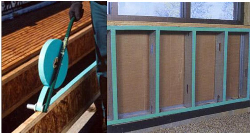
**Figure 6: Integrity™ Gasket forms a thermal break at external wall framed with metal studs to prevent "shadowing" on gypsum board and reduce sound transmission. (<http://www.integritygasket.com/oldgallery1.asp>)**
