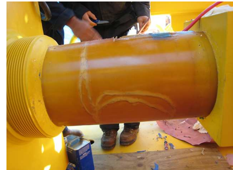
FIGURE 3. INSTALLATION ON THE MEASUREMENT STATION.
