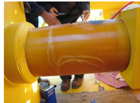
FIGURE 3. INSTALLATION ON THE MEASUREMENT STATION.
