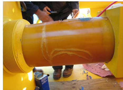
FIGURE 3. INSTALLATION ON THE MEASUREMENT STATION.
