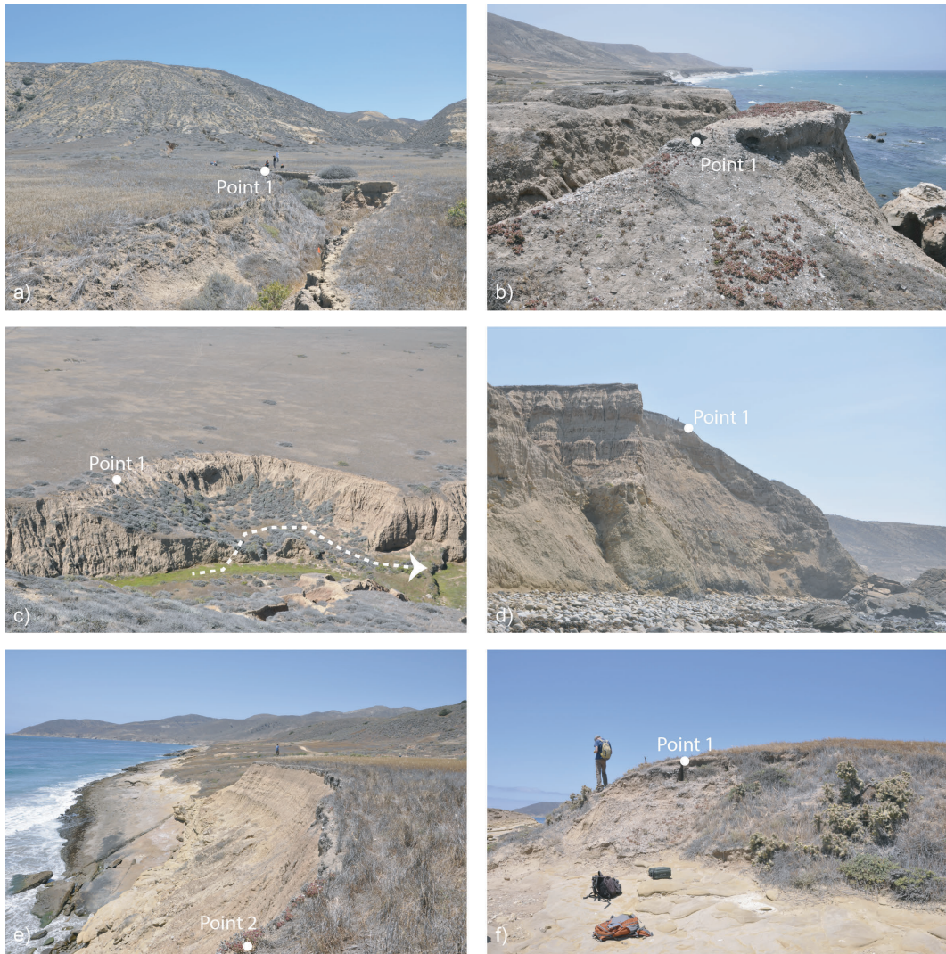
Fig. 8. Representative images of the types of erosion discussed in the text: (a) CA-SRI-333: A shallow gully cutting into the marine terrace; (b) CA-SRI-313: Remnants of a marine terrace dissected by gullies and eroding at the coast; (c) CA-SRI-338: The active channel of lower Bee Canyon formerly undercut this steep stream bank (see dotted arrow). Subsequent lateral migration and cutoff of a meander bend has moved the active channel away from this bank, leaving terraces at 2 elevations. A block of bedrock remains around which the stream used to flow; (d) CA-SRI-131: A steep sea cliff (approximately 30 m high) stands here. Cliff retreat is primarily caused by collapse of the whole terrace face, including weak bedrock and cap; (e) CA-SRI-138: Another example of sea cliff retreat, this time dominated by wave action below, with a collapse of the whole face; (f) CA-SRI-488: Another sea cliff at the marine terrace edge being eroded by waves below. In this close-up of the top edge of the terrace, the bedrock contact is exposed where other forces, likely dominated by wind erosion, have removed the terrace-capping sediment.
