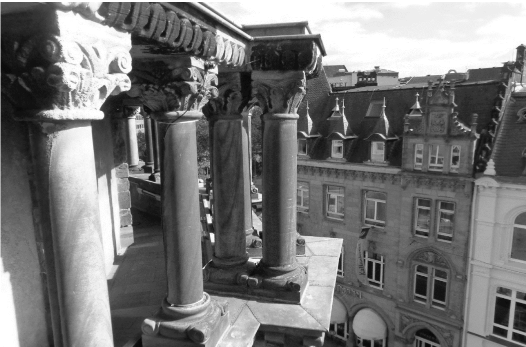
Trier – the city of many ages: a view from the ancient Roman city gates Porta Nigra – the oldest fortified structure in Germany. (Photo by the Author)
