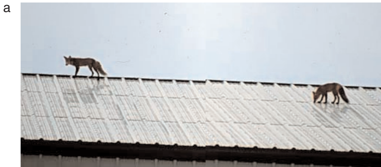
Fig. 1a. Red foxes on the sheet metal roof, 9.5 m aboveground.
