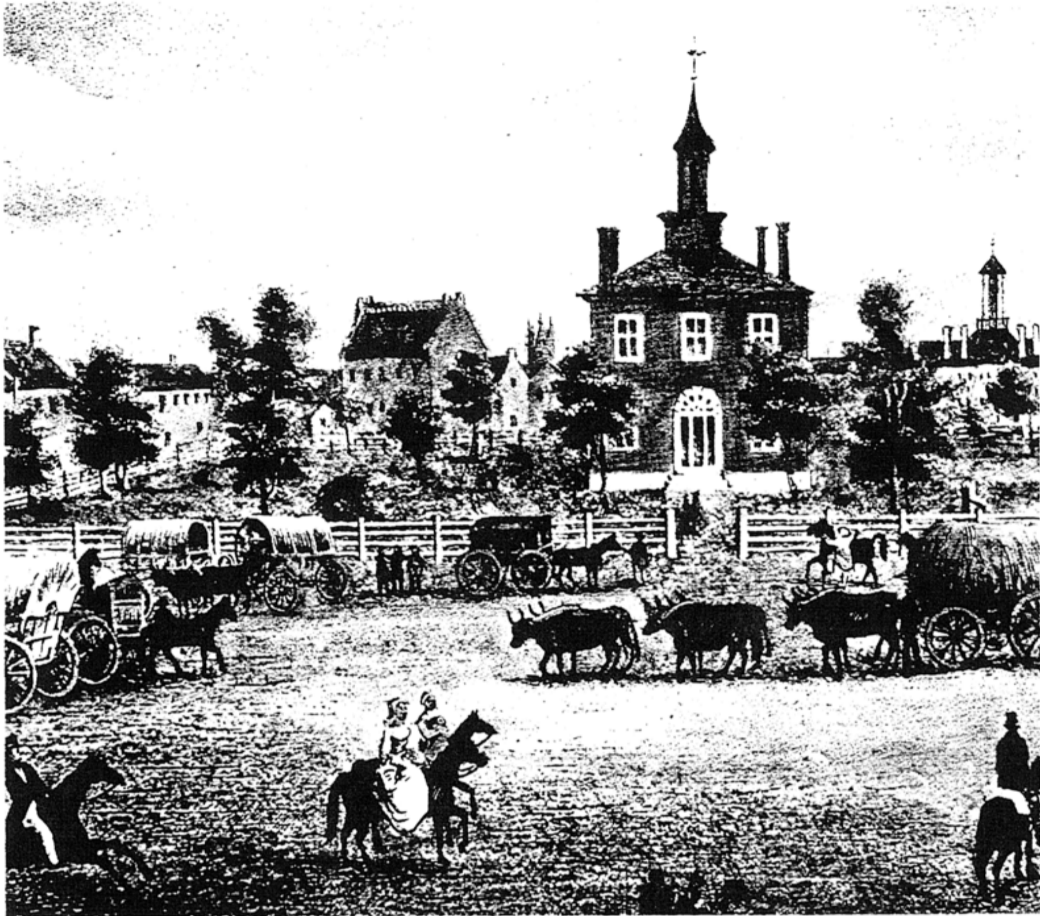
The second brick courthouse on the square in Independence, Missouri, as pictured by an unknown artist, c1850.
