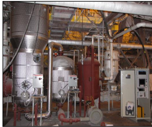
Figure 4: Flue Gas \text{CO}_2 Capture and Mineralize Pilot Process. (from right to left: Horiba flue gas analyzer, flue gas inlet, MDR, blower, humidifier, FBR).
