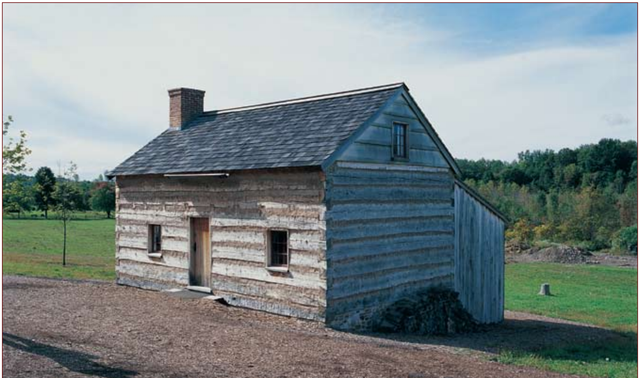
Shortly before Oliver left for Pennsylvania, the Smith family was forced to move back into the log home on their family farm. This replica of the log home stands on the site today. Courtesy IRI.
