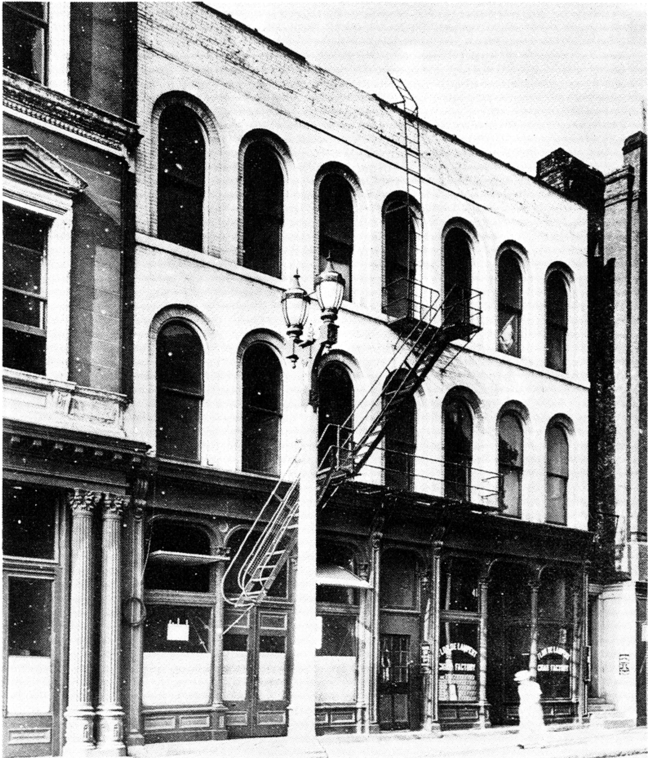
A St. Louis Dispatch file photo of Wyman's Hall prior to its destruction in 1941.
