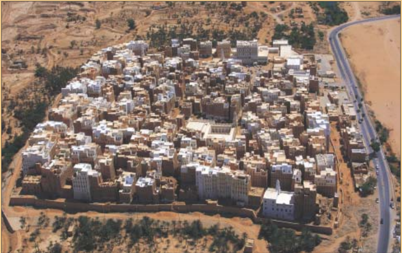
An aerial view of the skyscrapers of modern Shibam, in the Hadhramaut Valley of Yemen. Courtesy John J. Nowell and Zodiac Publishing.
