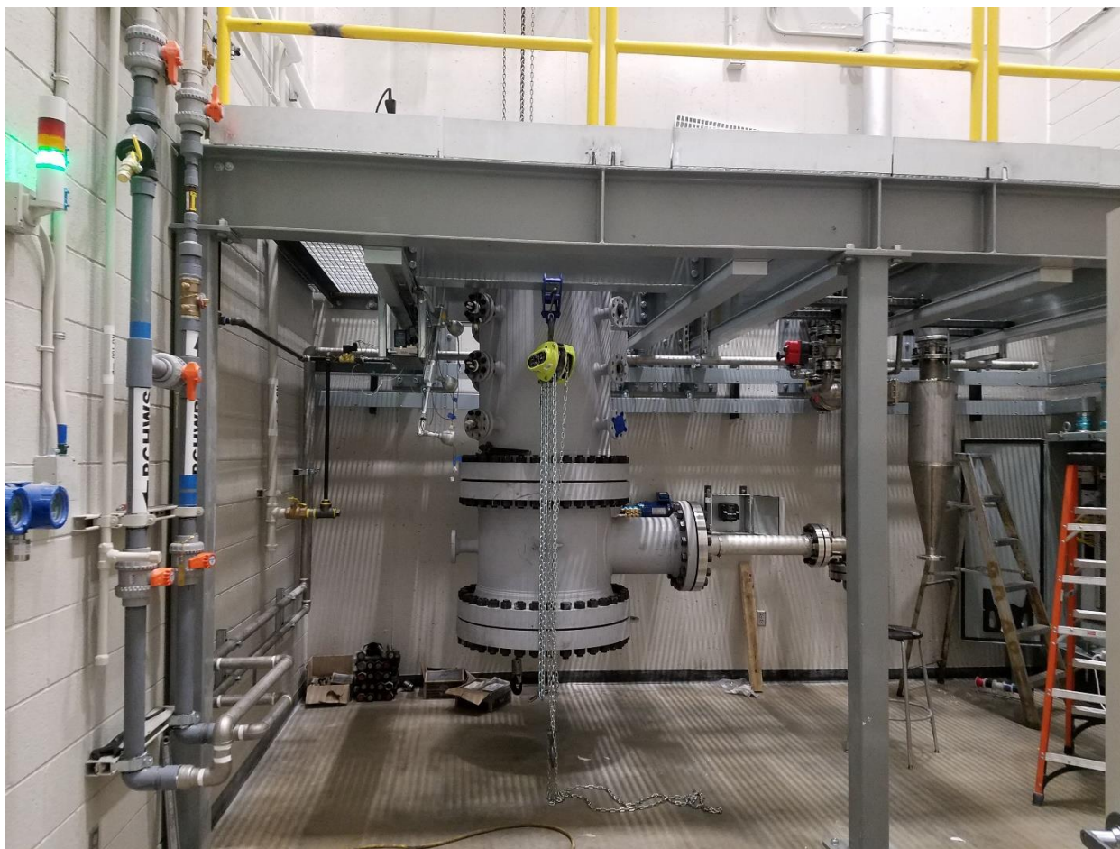
Figure 11. POC Reactor configured for atmospheric combustion.
