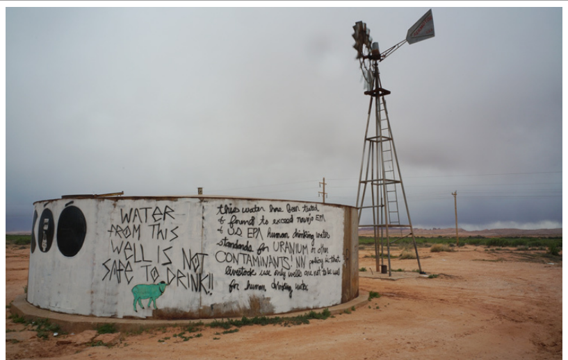
Figure 1. Photo of a contaminated well on the Navajo Nation. Groundwater and surface water were polluted with uranium, arsenic, and other heavy metals from widespread mining during the 20 th century.
