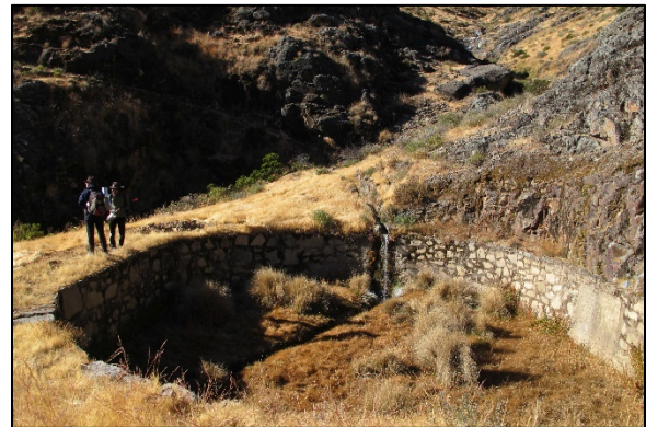
Figure 3.9. Stone and cement reservoir at the site of Puquio Sangre that collects rainwater and directs runoff from the quebrada (upper portion of photo). The reservoir has an intake canal (center) that picks up water from the quebrada and directs it into the basin. On the left is the outtake canal that connects to the Puquio Sangre/Huarmishcoto irrigation system feeding the village of Llancha. This photo was taken in August of 2017 during the dry season and the reservoir is largely empty and not feeding the canal.
