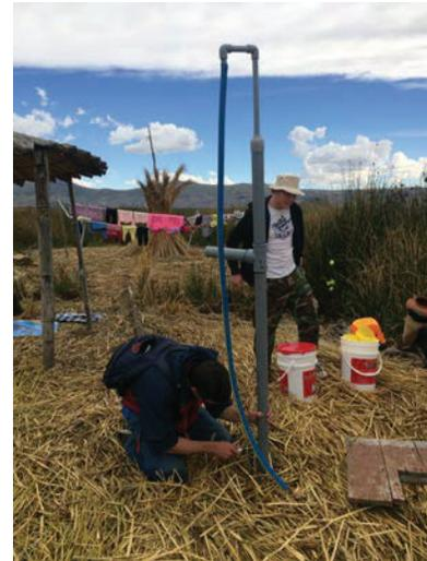
*Figure 3: Direct action lift pump being installed on the Uros Islands*
