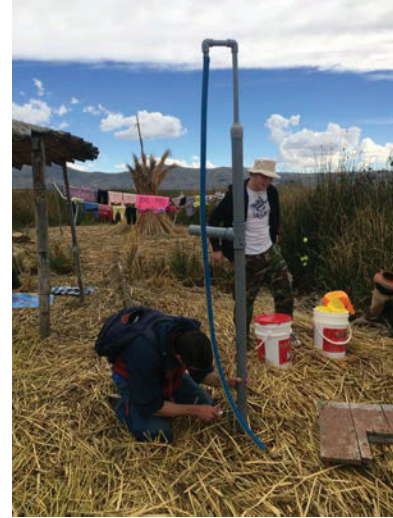
Figure 3: Direct action lift pump being installed on the Uros Islands
