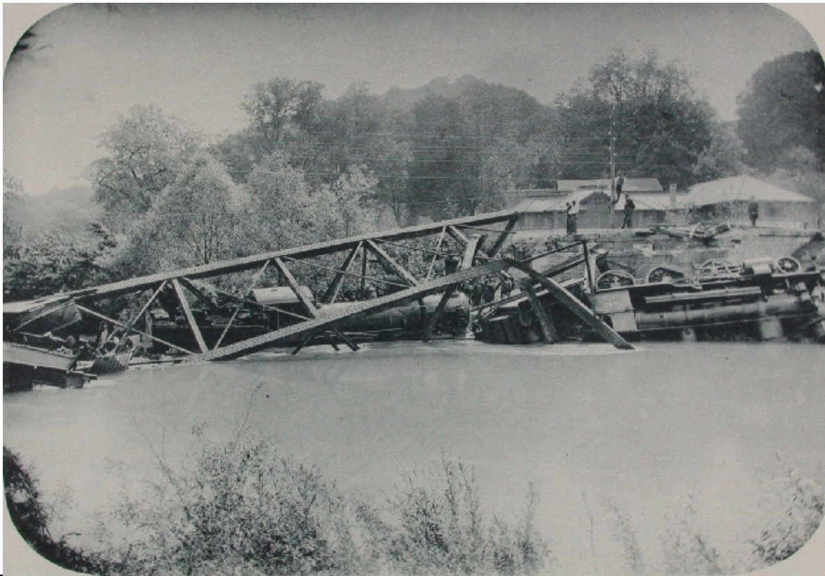
Figure 3 The Münchenstein train engines and bridge debris in the Birs
