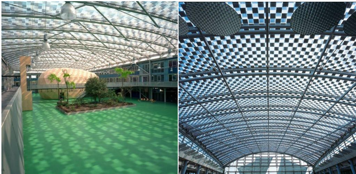
Figure 2-3 Variable shading ETFE foils used in the Kingsdale School in London, UK and Festo headquarters in Esslingen, Germany. (Vector Foiltec 2012)
