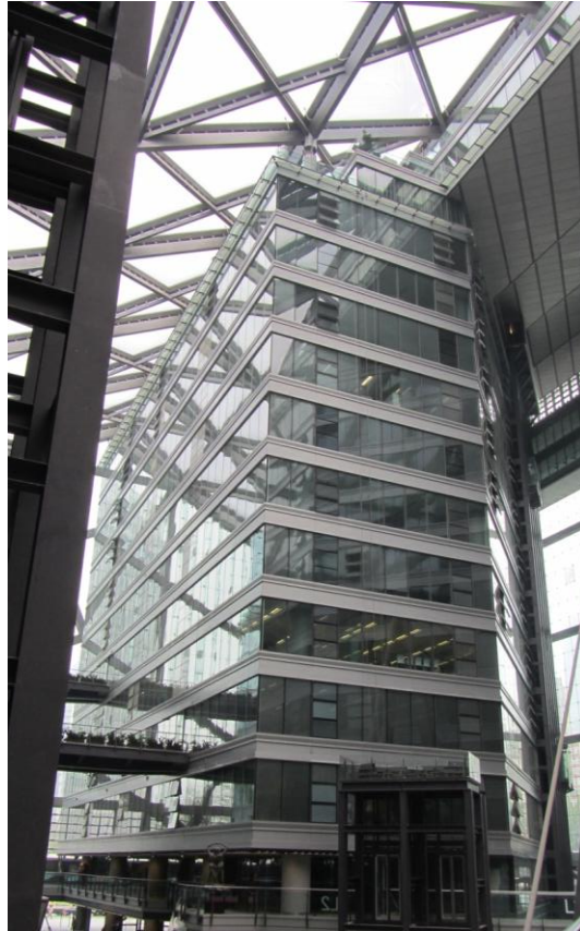
Figure 2-2 Parkview Green atrium with ETFE roof and glass walls
