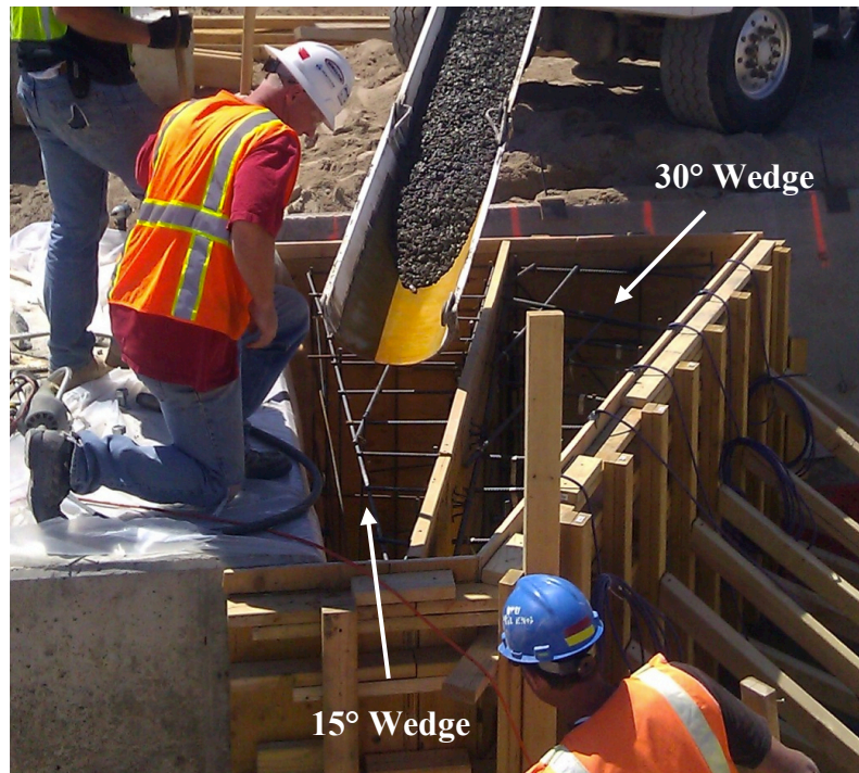
Figure 3-4: Casting of 15° and 30° wedges
