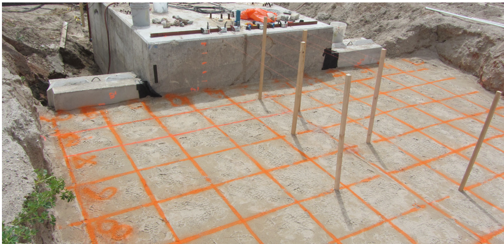
Figure 3-34: Backfill surface fully prepped for testing
