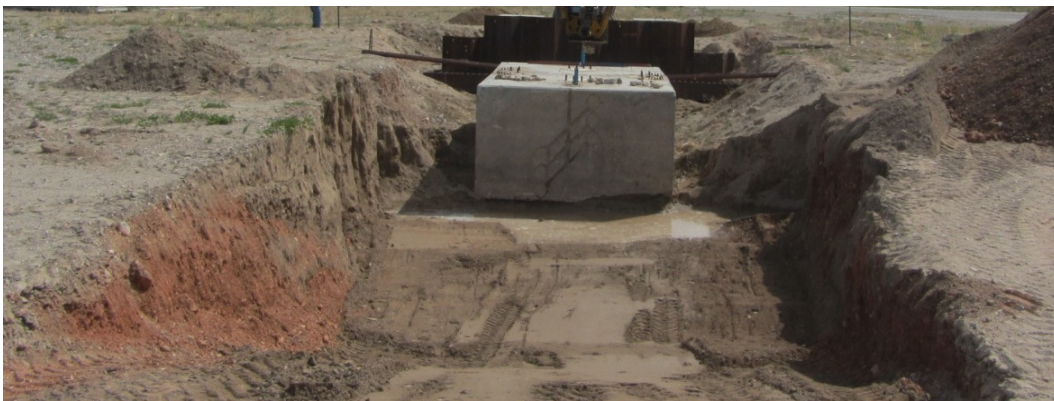
Figure 3.12: Test site backfill zone
