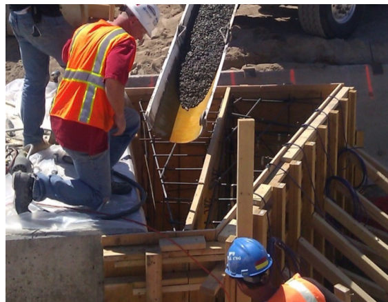
Figure 3.10: Construction of 15° and 30° wedges (Marsh 2013)
