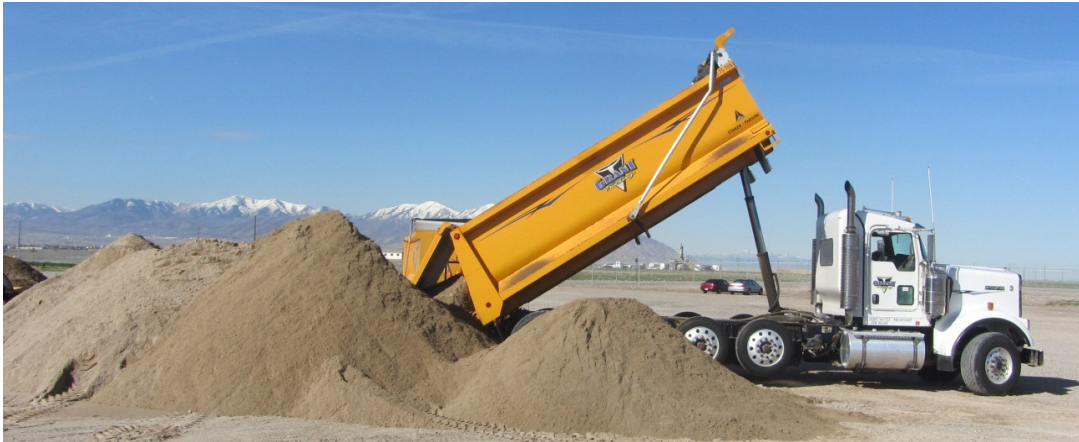
Figure 3.13: Delivered backfill sand (SP)
