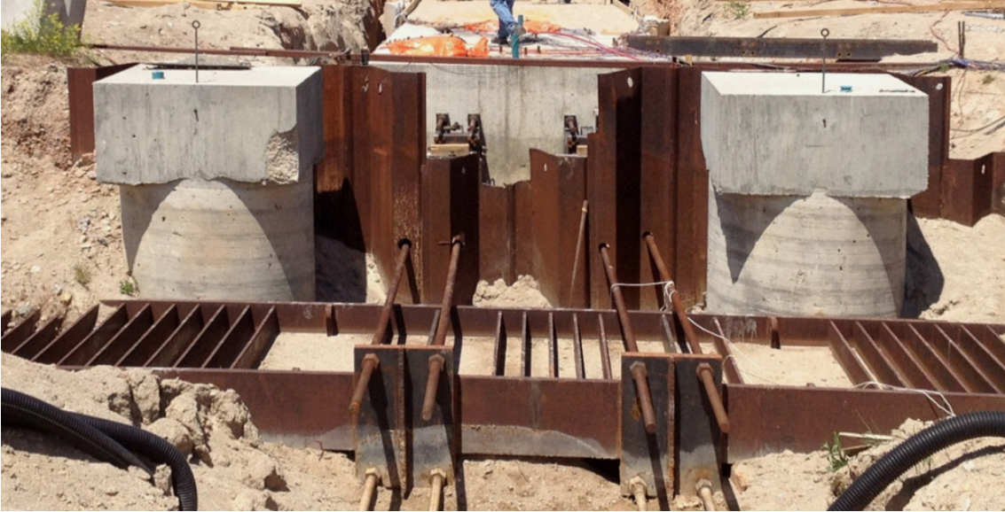
Figure 3.7: South side of reaction foundation
