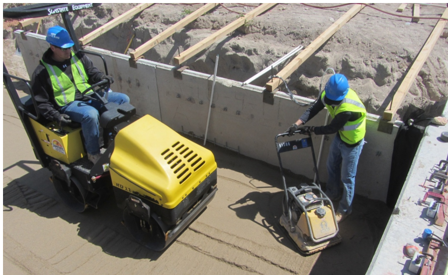
Figure 3.28: Compaction instruments with vibrator roller compactor on left and plate compactor on right
