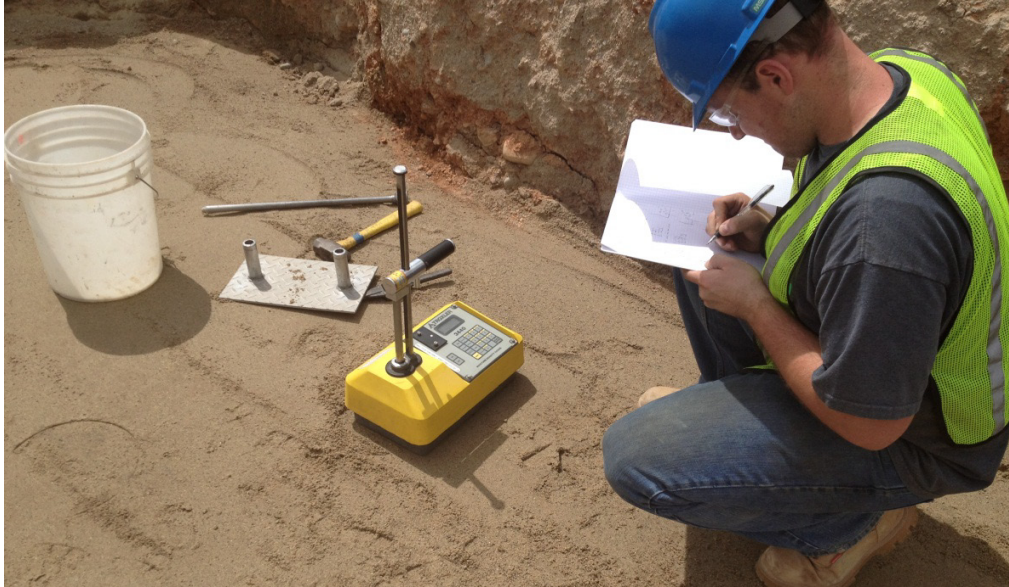
Figure 3.29: Testing soil with nuclear gage
