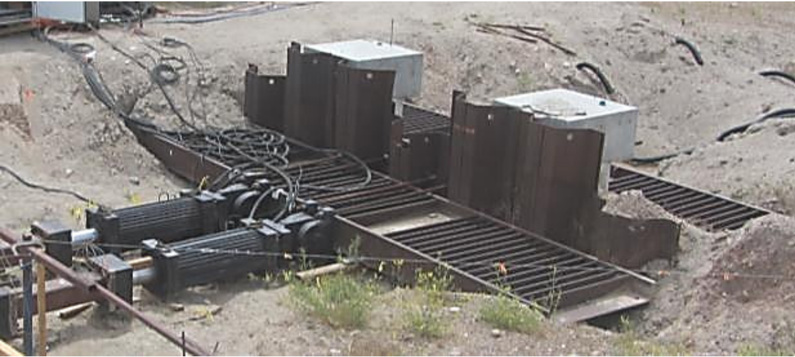
Figure 3.8: North side of reaction foundation
