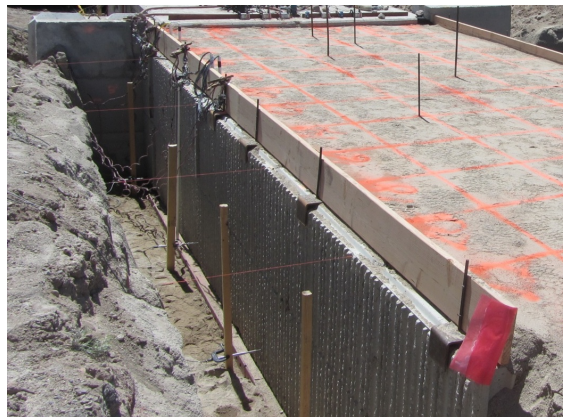
Figure 3.25: MSE wall instrumentation setup for 0° test
