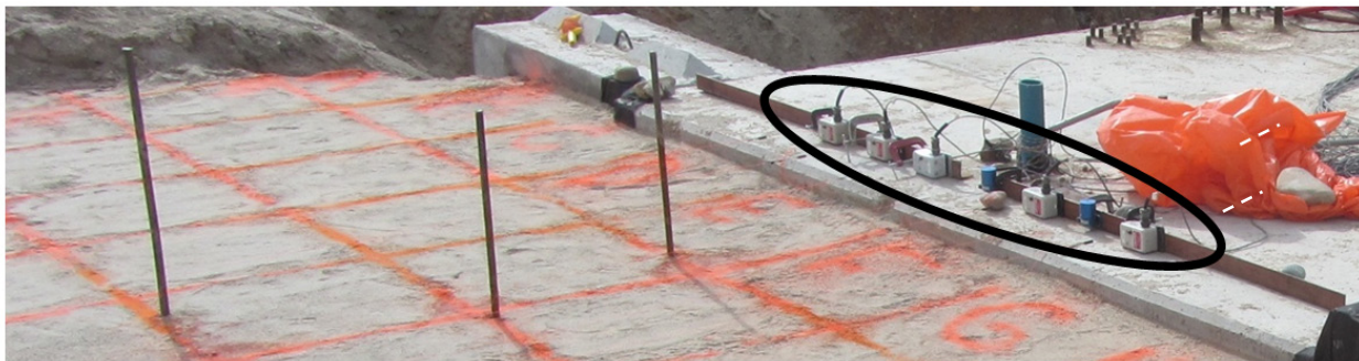
Figure 3.24: String pot arrangement for zero skew backfill deflection measurements
