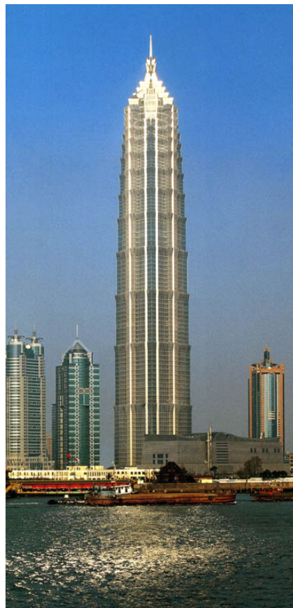
Figure 1-1: Jin Mao Tower – Shanghai, China © SOM
