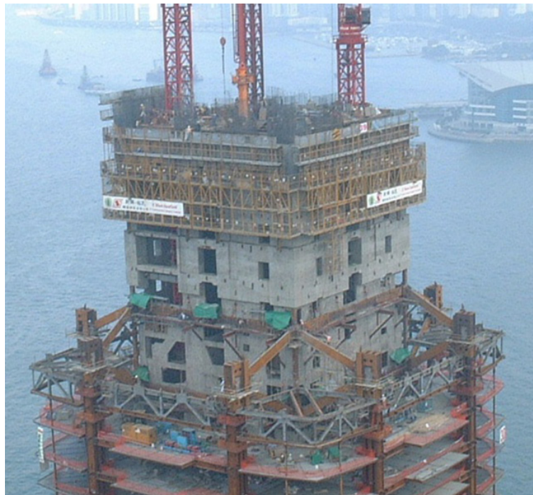
Figure 1-6: IFC2 - typical layout of outrigger and belt trusses (Emporis.com)
