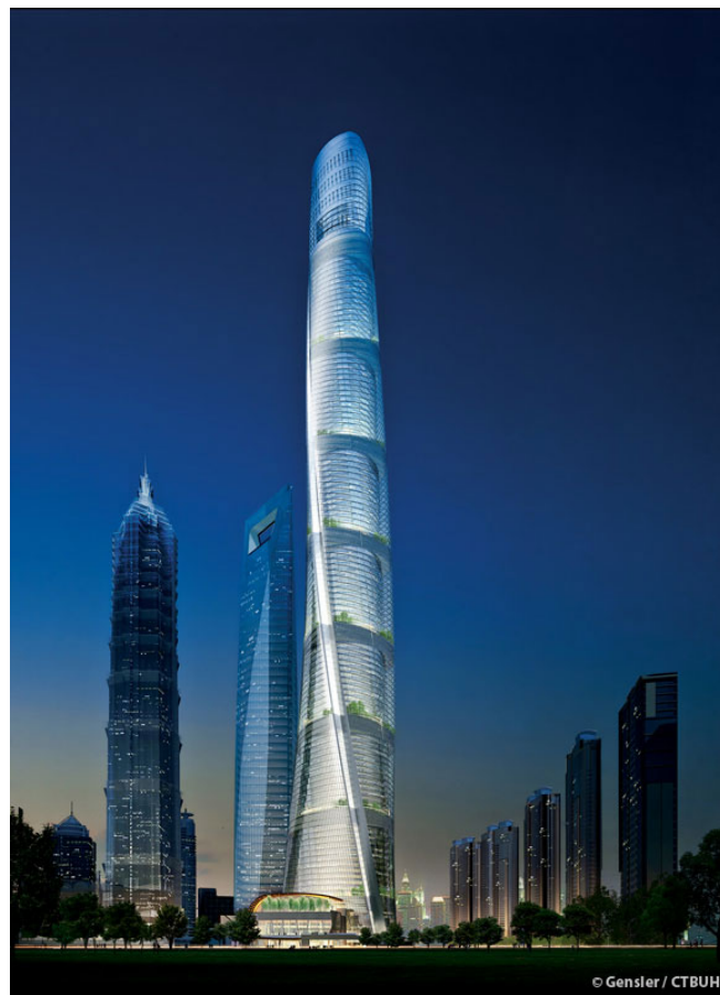
Figure 1-7: Shanghai Tower © Gensler
