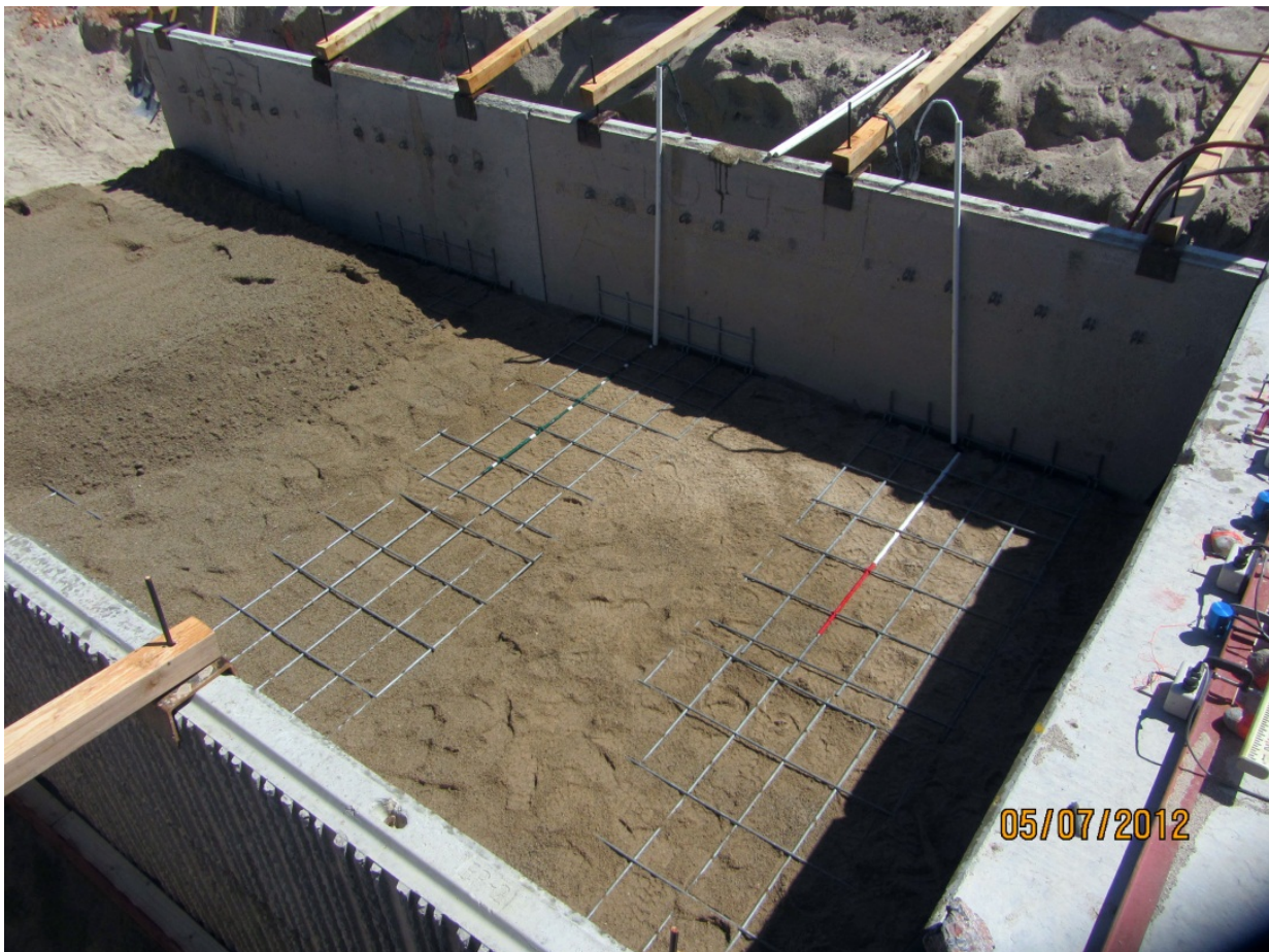
Figure 3.18: Installation of the Instrumented Reinforcement Grids for the Zero Skew Test
