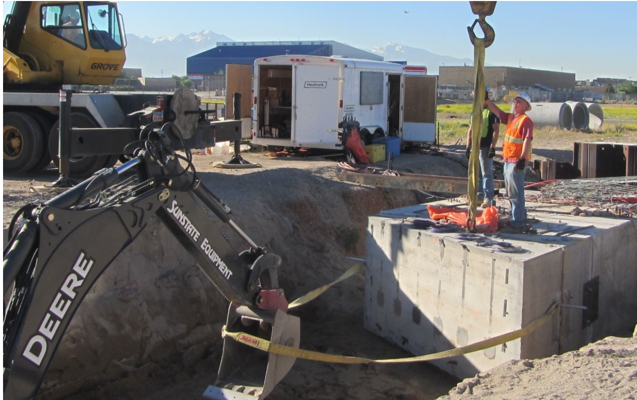
Figure 3.12: Removal of the 30° Concrete Wedge
