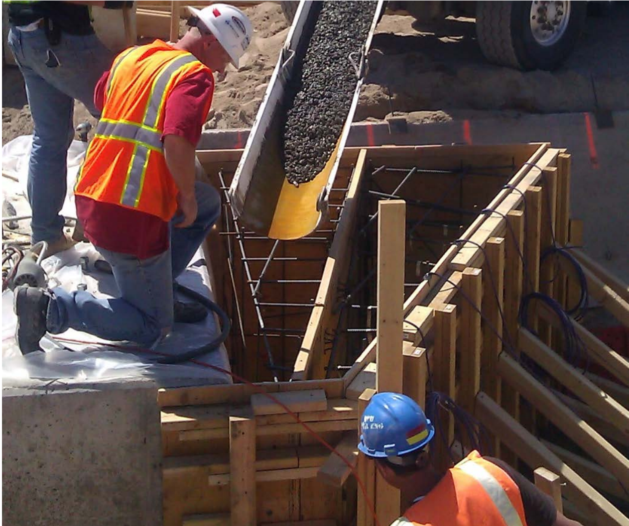
Figure 3.6: Simultaneous Casing of the 15° and 30° Wedges
