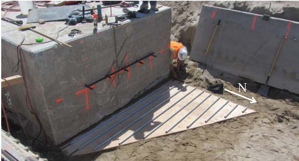
Figure 3.11: Steel Roller Bearing Platform for Concrete Wedges
