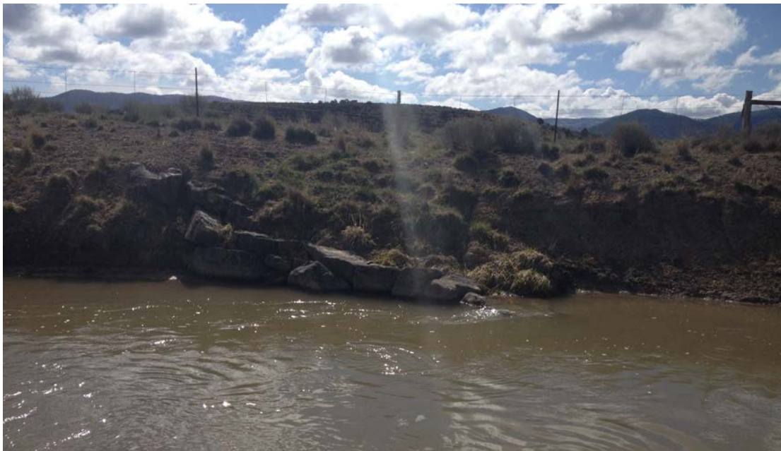
Figure 3-9: Steep Vane Slope has Increased Steambank Erosion. Flow from Right to Left. (Picture Taken by Evan Cope)
