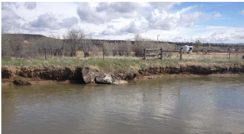
Figure 3-5: Large Vane Angle that Created a Recirculating Eddy and has Actually Increased Streambank Erosion. Flow from Right to Left. (Picture taken by Evan Cope).
