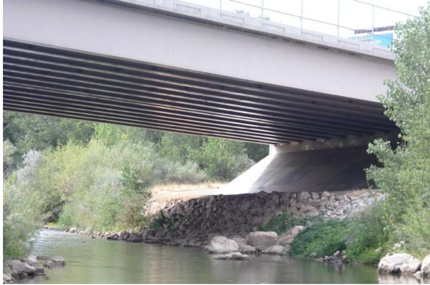
Figure 2-3: Riprap Used to Protect a Bridge Abutment. Flow From Top to Bottom (Picture Taken by Evan Cope).
