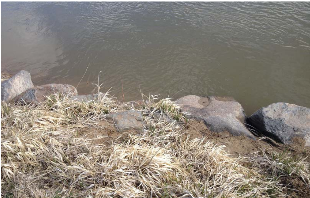
Figure 3-7: Tight Vane Angle Protected and Stabilized the Streambank. Flow from Right to Left (Picture Taken by Evan Cope).
