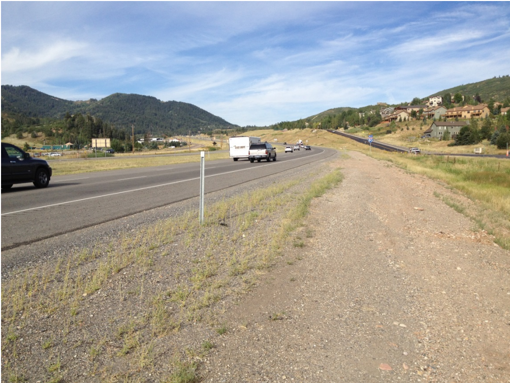
Figure 6-8: Typical shoulder on Interstate 80.
