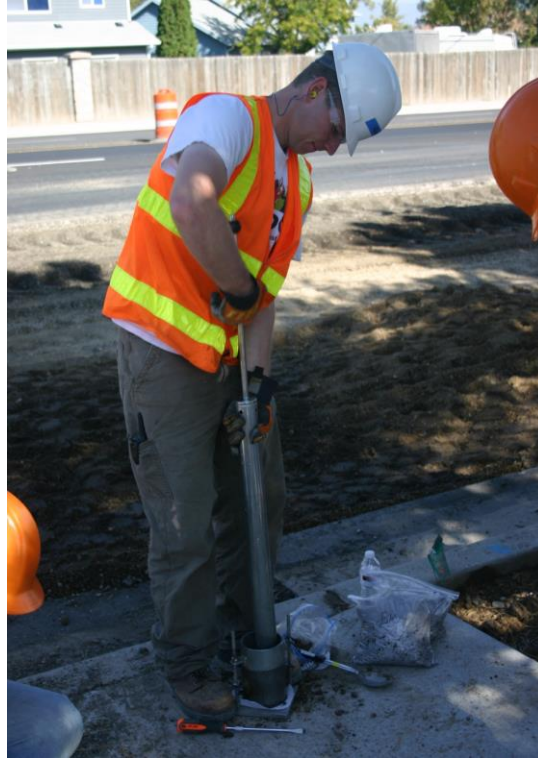
Figure 3-3: Compaction of emulsion-treated base specimen at 7800 South.
