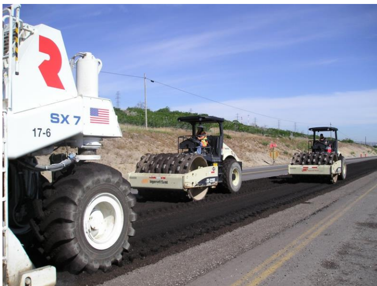
Figure 2-3: Compaction of emulsion-treated base layer at Redwood Road.
