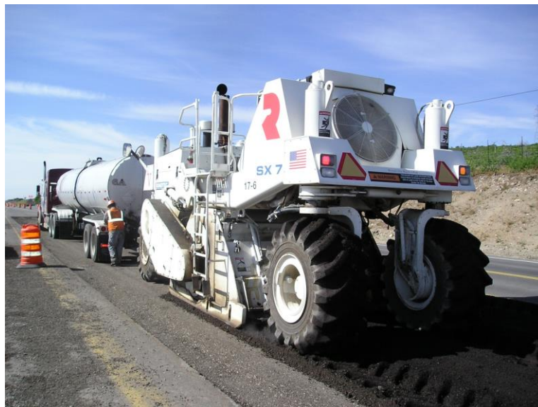
Figure 2-1: Asphalt emulsion injection at Redwood Road.
