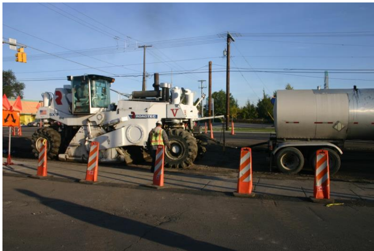
Figure 2-2: Asphalt emulsion injection at 7800 South.
