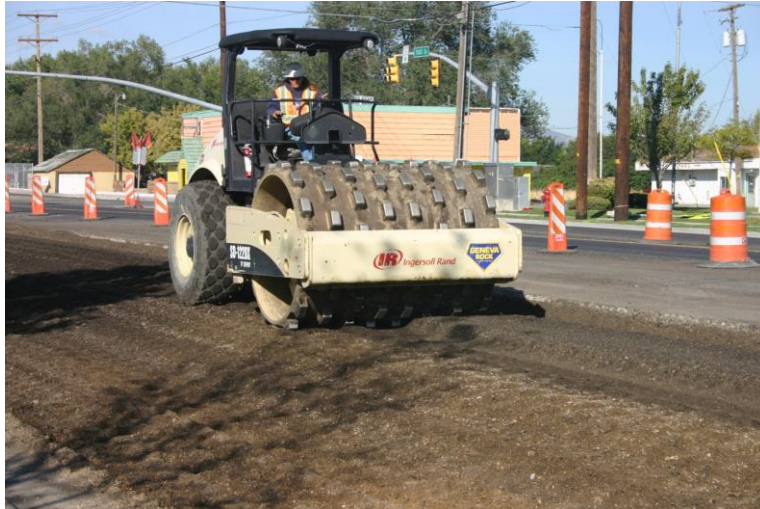
Figure 2-4: Compaction of emulsion-treated base layer at 7800 South.
