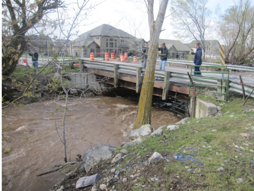
Figure A.3: Sampling from a culvert upstream of middle site
