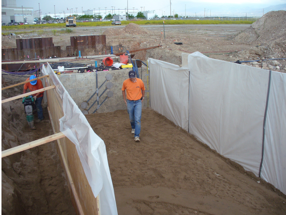
Figure 4-8: Picture of side isolation panels being backfilled.
