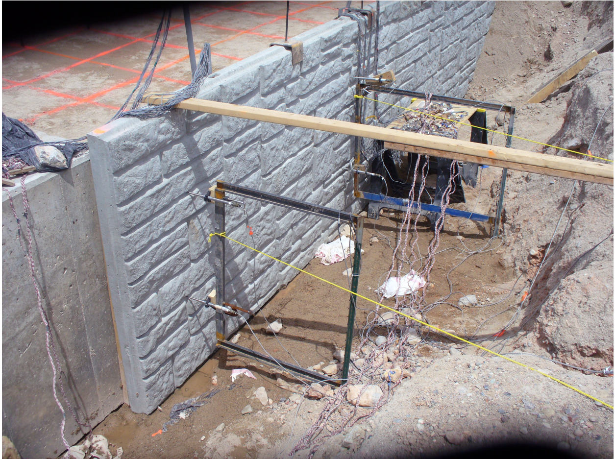
Figure 4-18: LVDT's to measure wall deflection.
