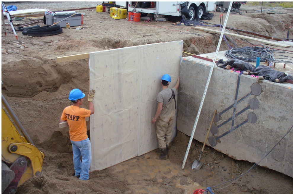
Figure 4-7: Installation of side isolation panels.
