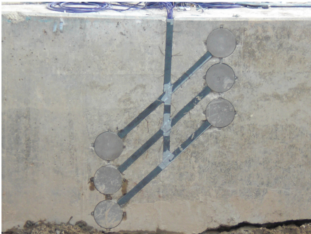
Figure 4-4: Pressure plates installed in the front face of the pile cap.
