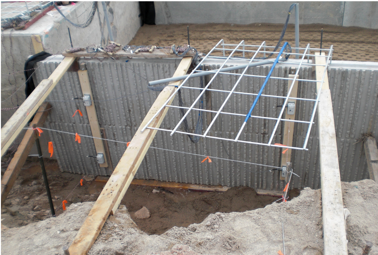
Figure 4-15: String pots to measure wall deflection.
