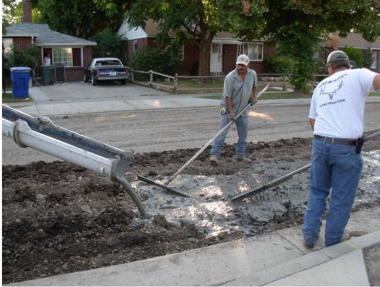
Figure 2-2: Cement slurry application directly from a truck chute.
