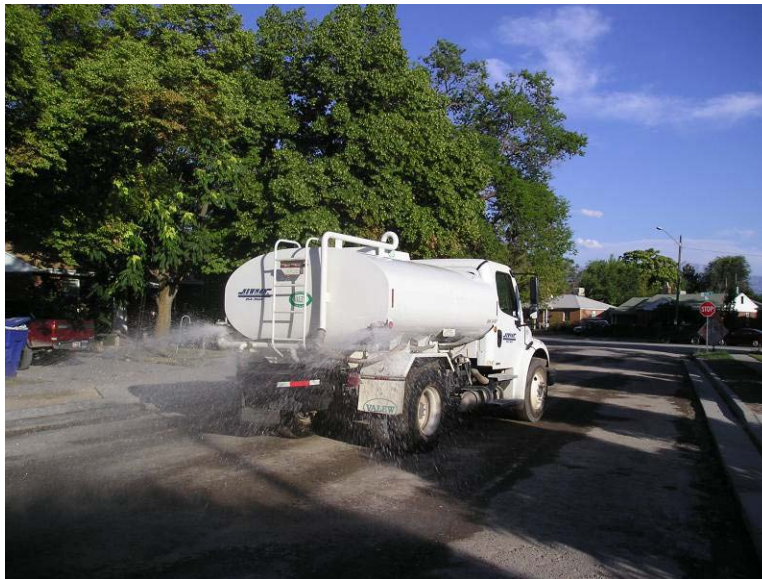
Figure 2-5: Moist curing using a water truck.
