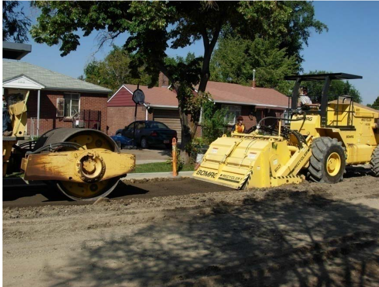
Figure 3-10: Mixing and compacting CTB layer.
