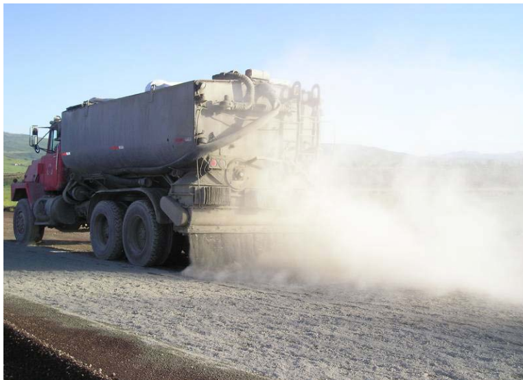
Figure 2-1: Cement powder application.
