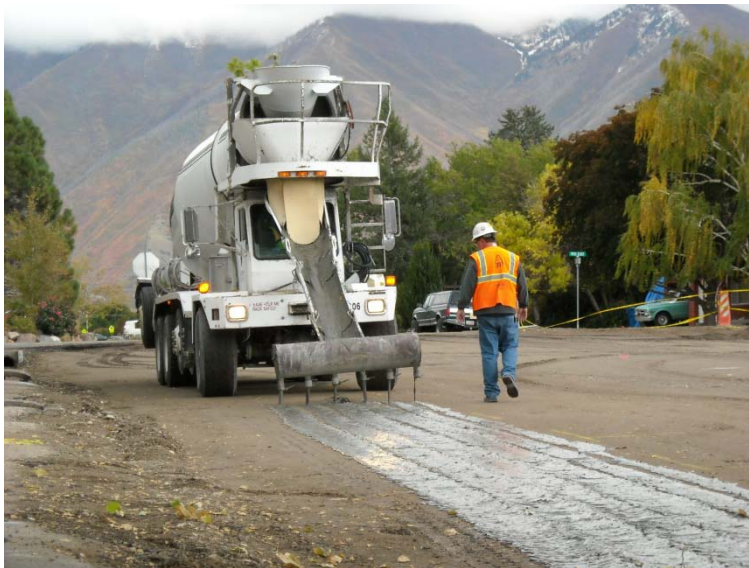
Figure 2-3: Cement slurry application using a cement slurry spreader.
