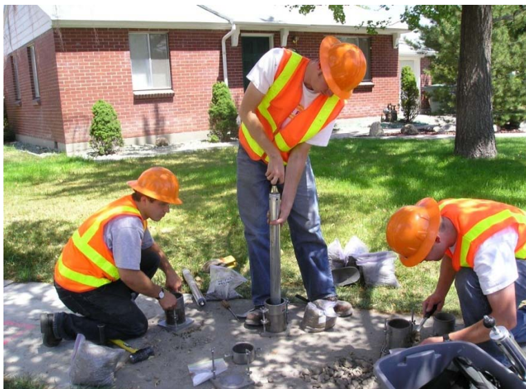
Figure 3-9: Compacting field specimens.
