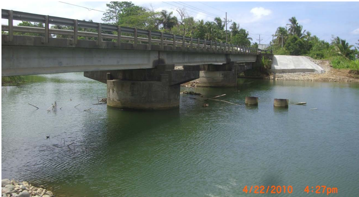
Figure 10-1: The Current Rio Bananito Highway Bridge
