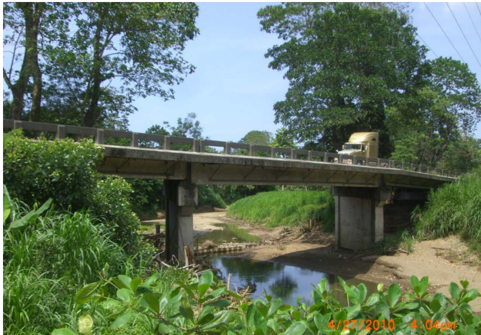
Figure 9-1: The Rio Blanco Bridge
