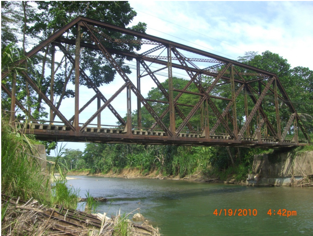
Figure 11-1: The Rio Bananito Railway Bridge
