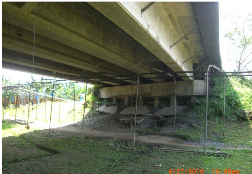
Figure 8-1: The East Abutment of the Rio Cuba Bridge
