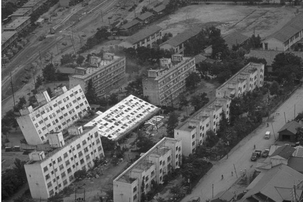
Figure 2-14: Bearing Capacity Failures Following 1964 Niigata, Japan Earthquake (Courtesy of EERC, Univ. of Calif.)
