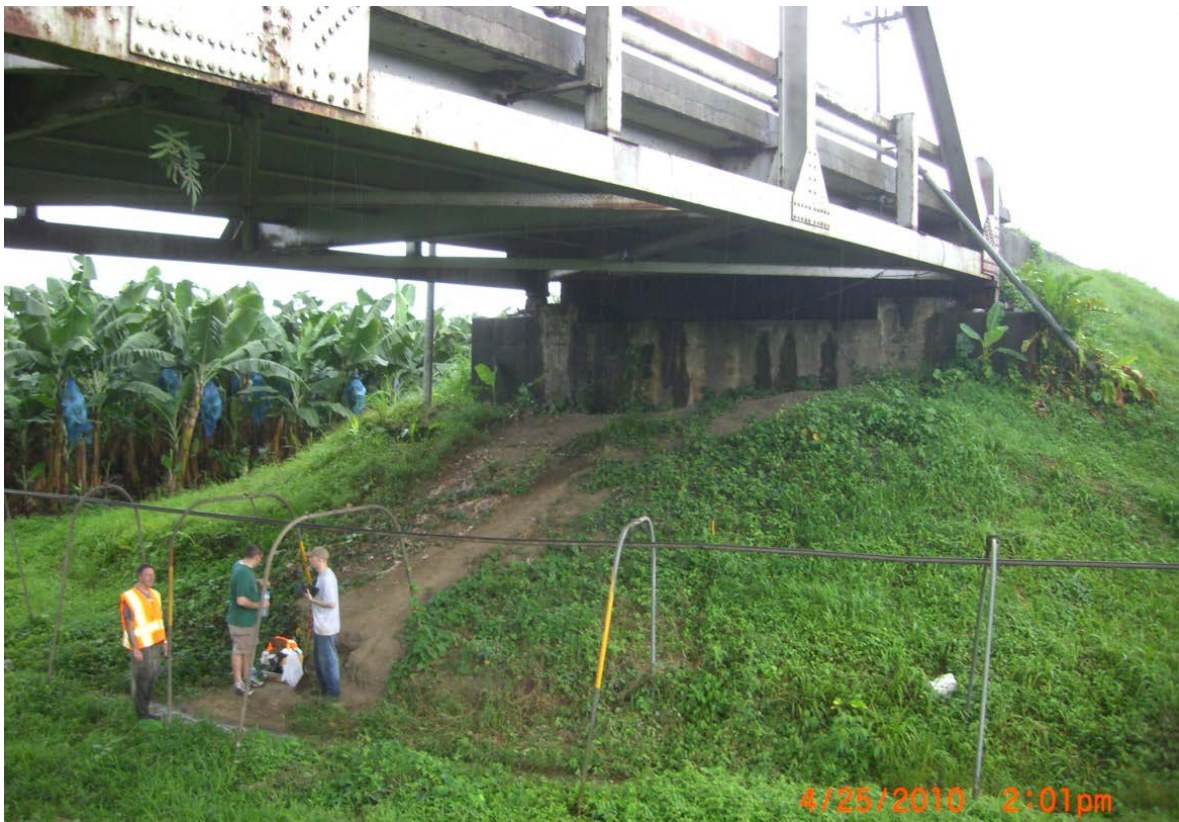
Figure 12-1: Southern Abutment of the Rio Estrella Bridge
