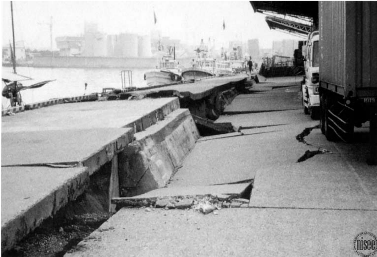
Figure 2-15: Graben Formed Behind a Displaced Quay Wall in Kobe, Japan Following 1995 Hyogoken-Nanbu Earthquake (Courtesy of NISEE, Univ. of Calif.)
