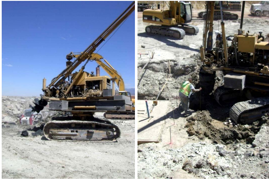
Figure 5-7 Excavation for RAP installation
