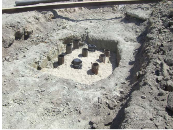
Figure 4-3 Driven pile layout prior to cap construction
