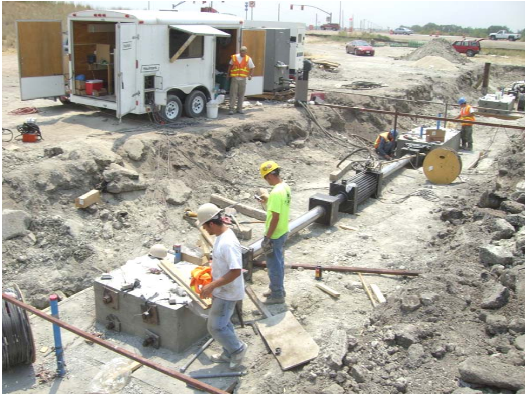
Figure 4-9 Photo of actuator setup between caps 1 & 2
