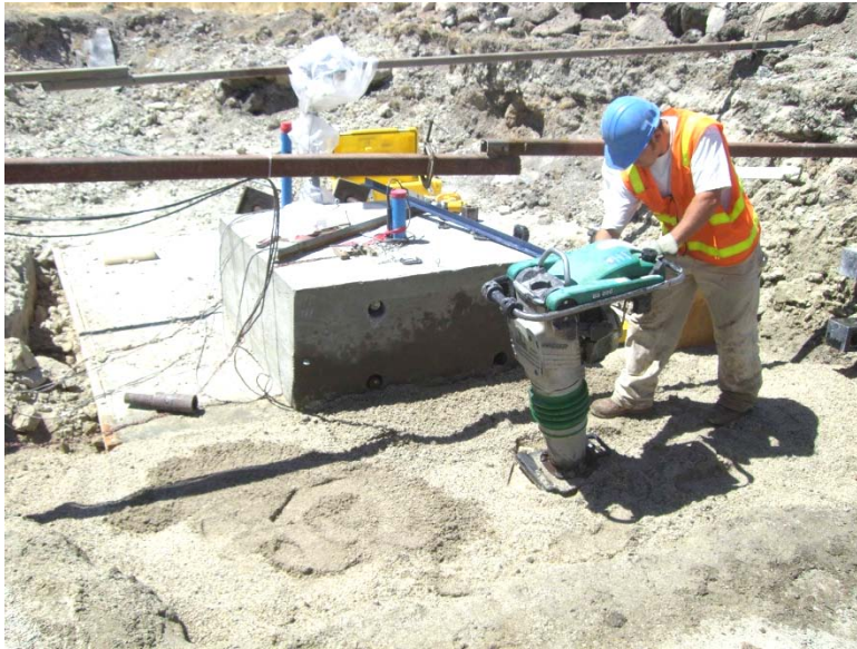
Figure 5-3 Passive resistance region of compacted sand fill being compacted
