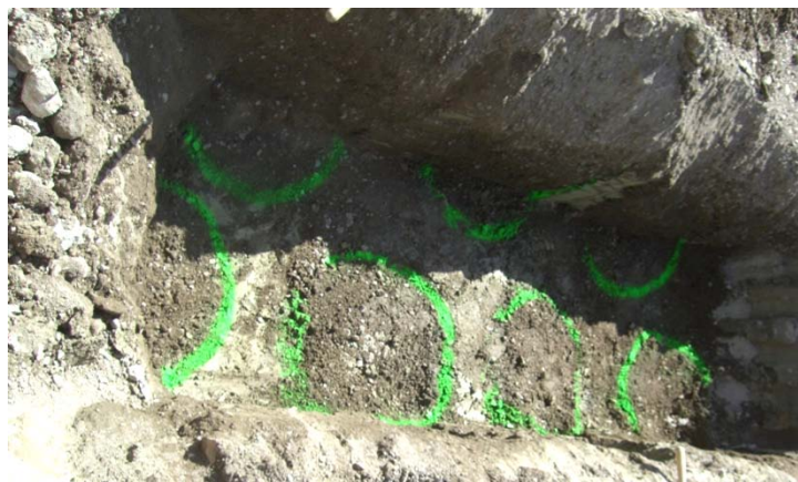
Figure 1-13 Photo of finished excavation with the RAP columns highlighted
