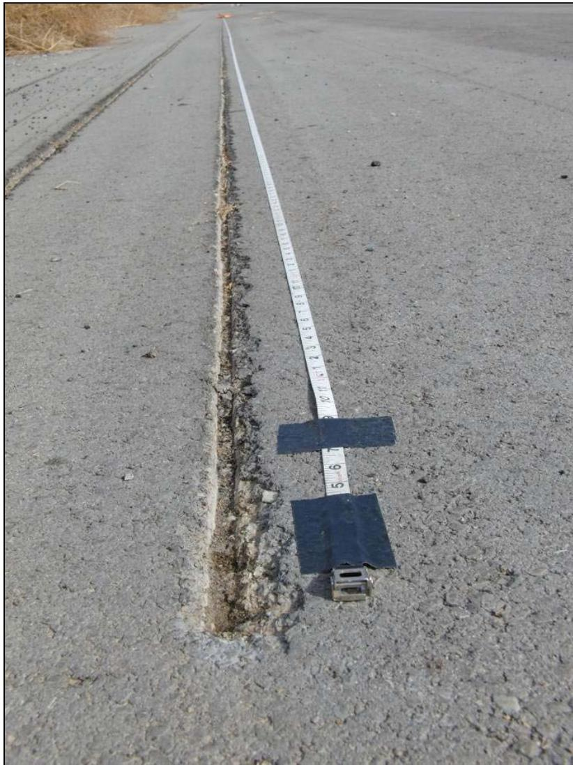
**Figure 3.3 Tape measure next to gouge**
