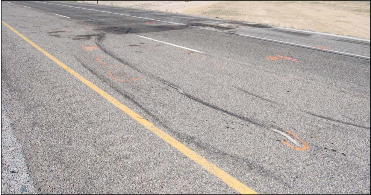
**Figure 2.2 Example of a roadway gouge caused by a wheel rim**
