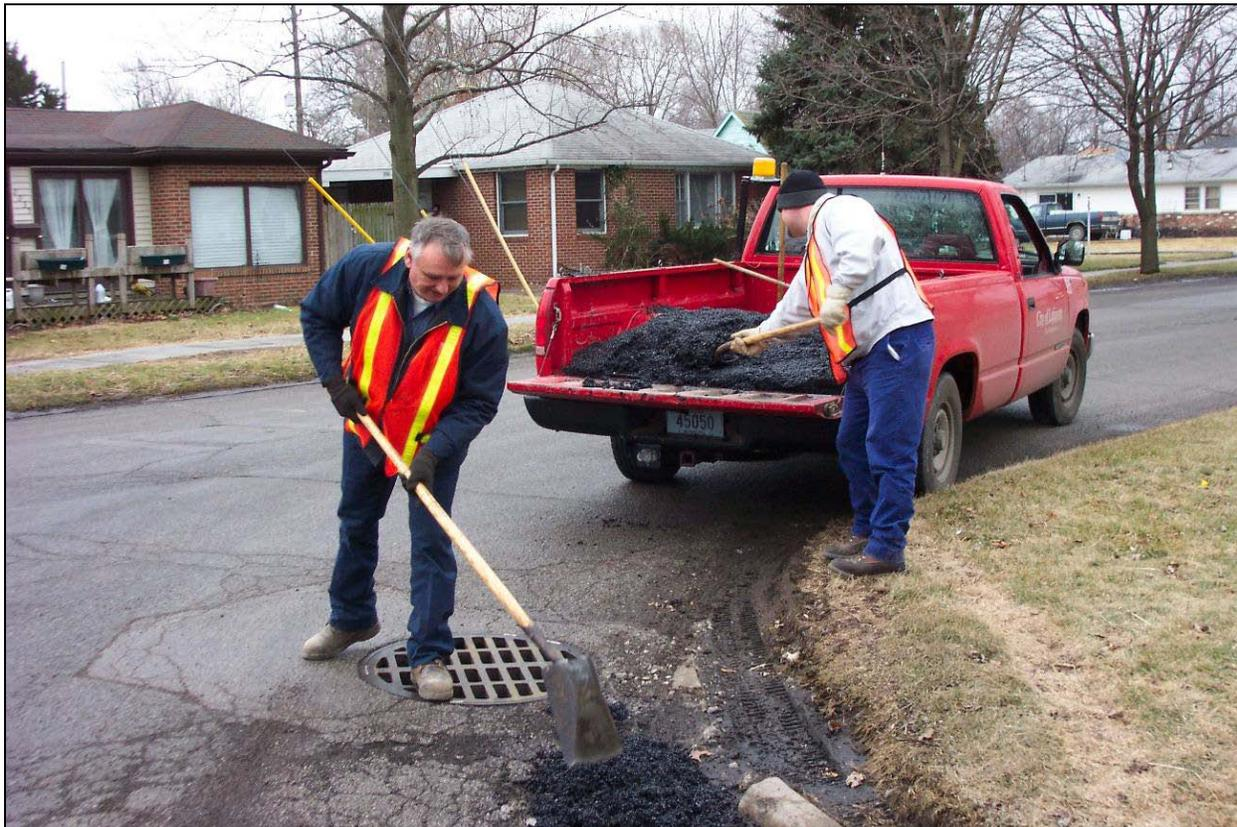
Figure 2.5 Example of cold mix asphalt patching [Layfayette]
