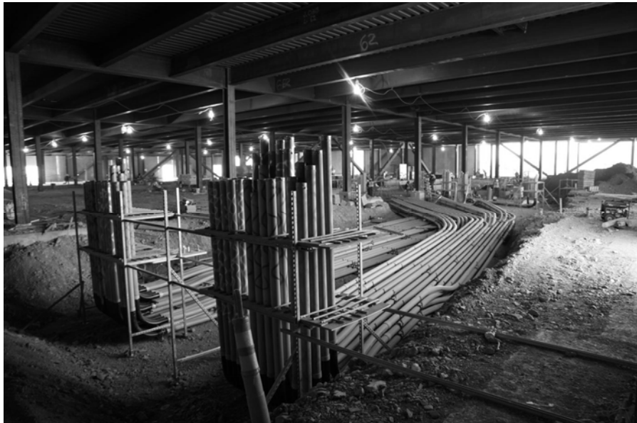
Figure 3.1.1: Underground Conduit in Data Center Construction
