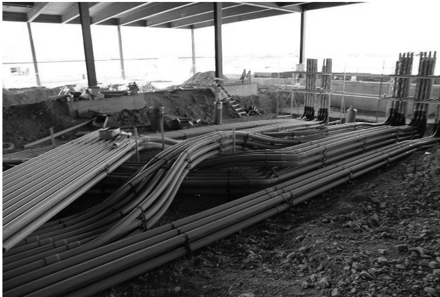
Figure 3.1.2: Underground PVC Conduit in Data Center Construction
