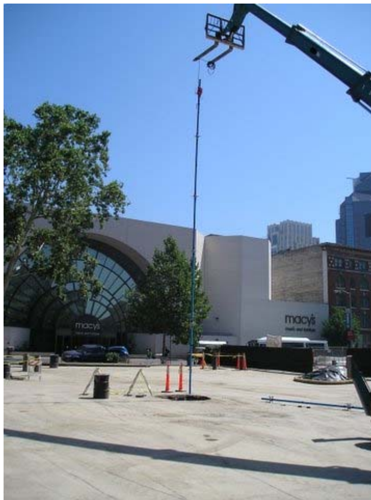
Figure 4-9 Installing Multiple Sections using Forklift in Sacramento, CA (author photo)
