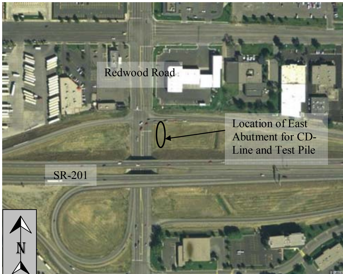
Figure 3-2 Aerial Photo of Redwood Road and SR-201 Site before Construction with Location of Test Pile (USGS, 2003)
