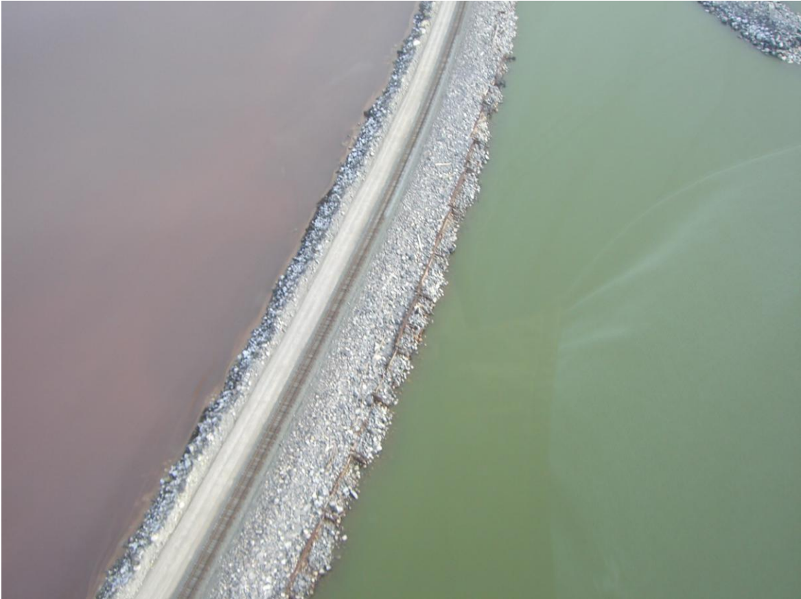
Figure 3: North and south sides of the railway causeway.
