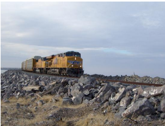
Figure 1: Union Pacific train on railway causeway
