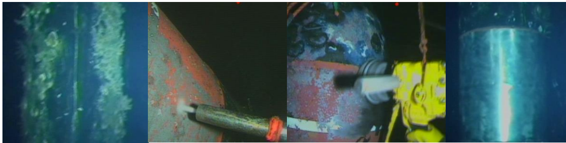
Figure 8. Tendon Preparation for Adhesive Clamp Bonding.
