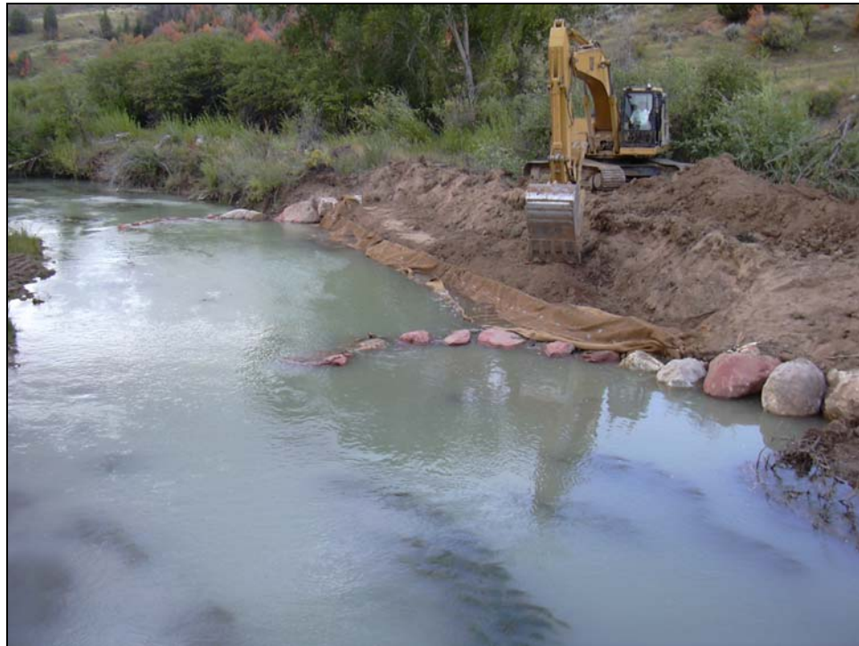
Figure 3-6. View of Construction From Bridge.
