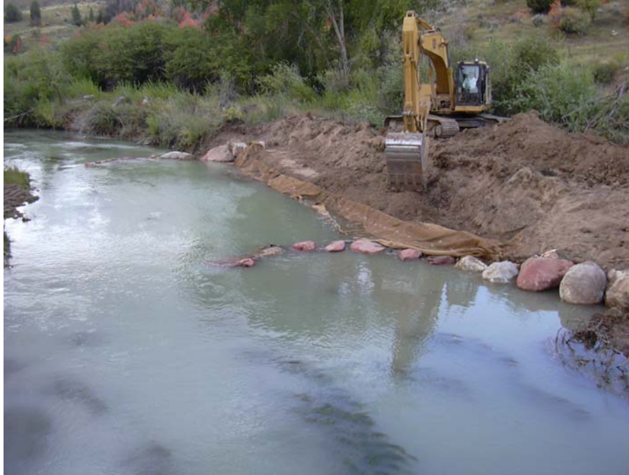
Figure 2-7. J-Hook Vane on the Spanish Fork River.
