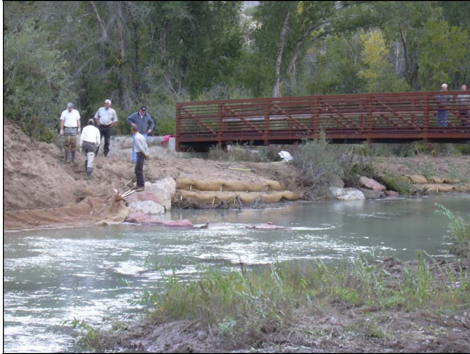
Figure 3-5. View of Construction of Structure Near Footbridge.
