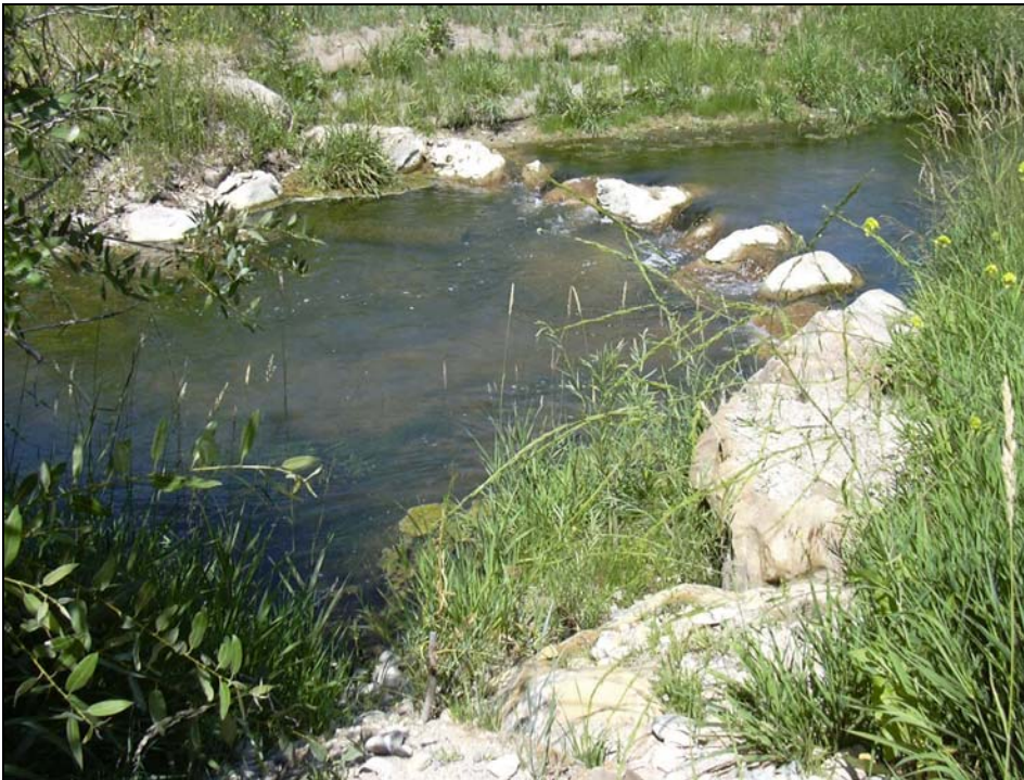
Figure 2-2. Porous Weir on the San Pitch River.
