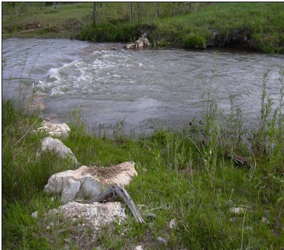
Figure 3-17. Cross-Vane Photo Taken During Spring Runoff 2004.
