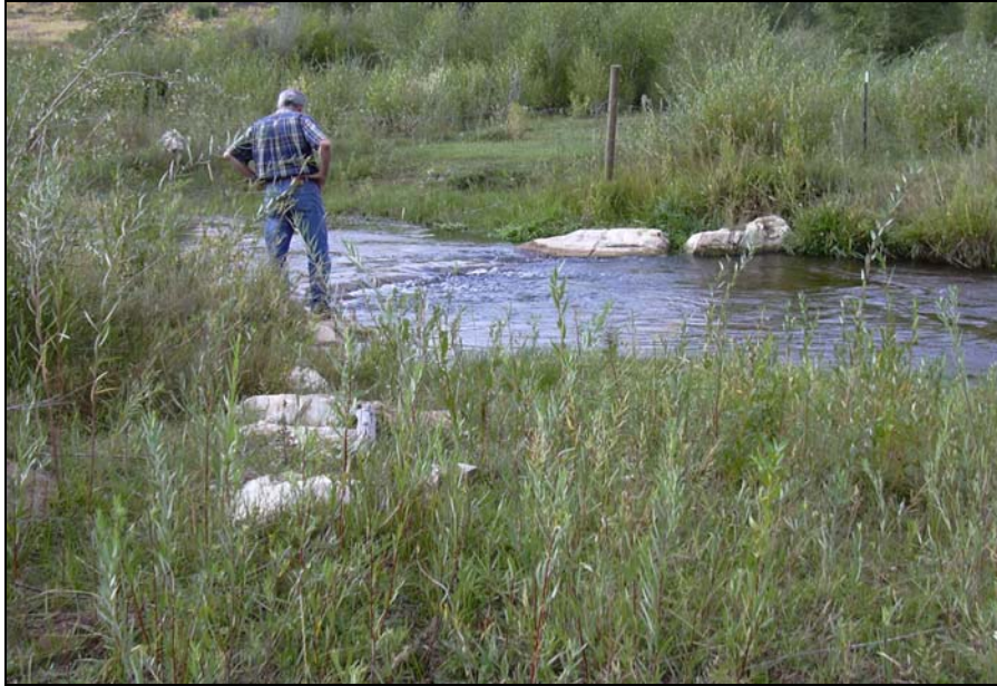
Figure 3-16. Cross-Vane Photo Taken Before Spring Runoff 2004.
