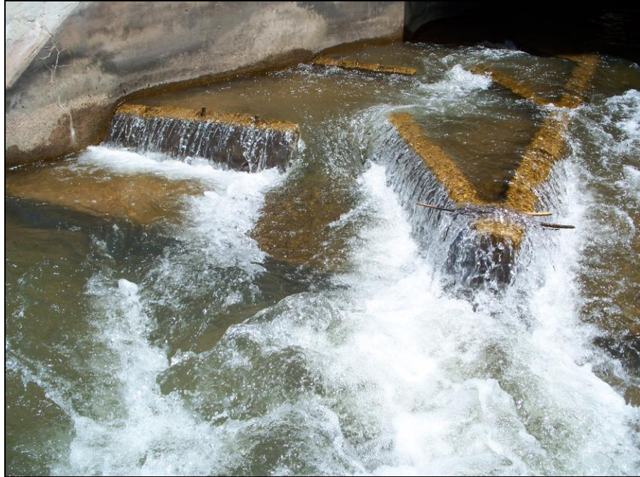
Figure 5-11: Photo at Outlet of Fish Baffles
