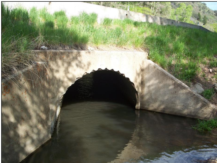
Figure 4-13: Outlet of Backwatered Culvert #3
