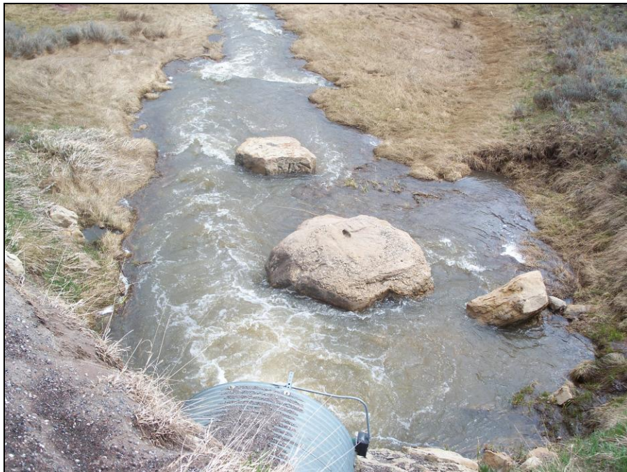
Figure 5-20: Large Boulders Downstream of a Culvert Outlet
