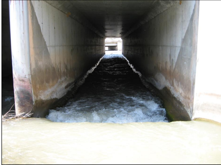
Figure 5-15: Spillway at Inlet
