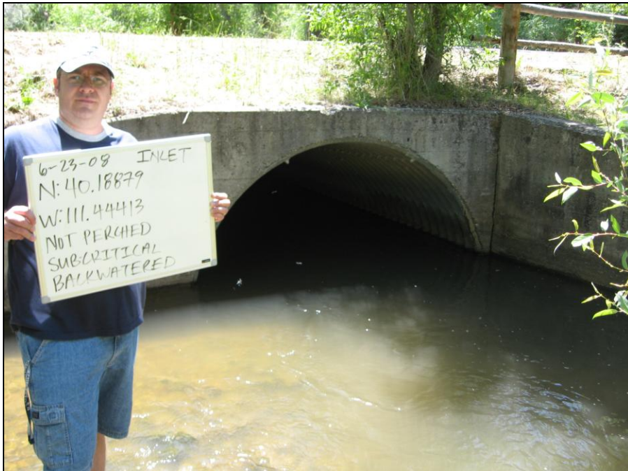
Figure 3-4: Hydraulic Evaluation Photo of a Culvert Inlet
