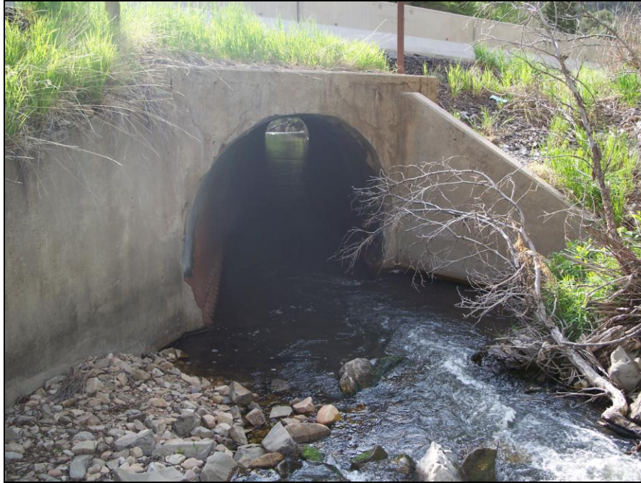
Figure 4-12: Inlet of Backwatered Culvert #3
