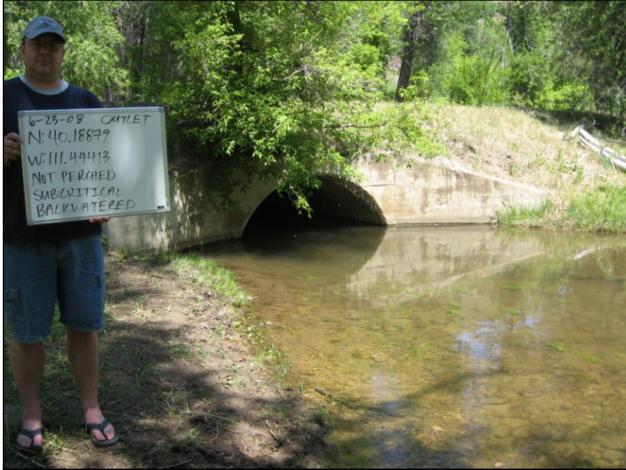
Figure 3-3: Hydraulic Evaluation Photo of a Culvert Outlet
