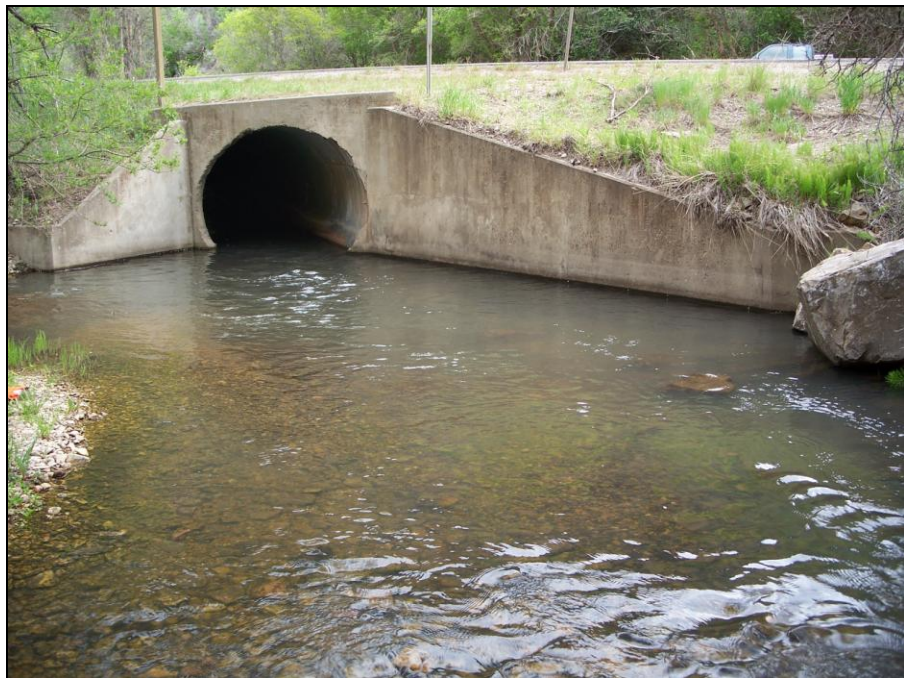
Figure 6-13: Daniel's Creek Culvert #2 Outlet (Daniels Creek Field Verification Site)
