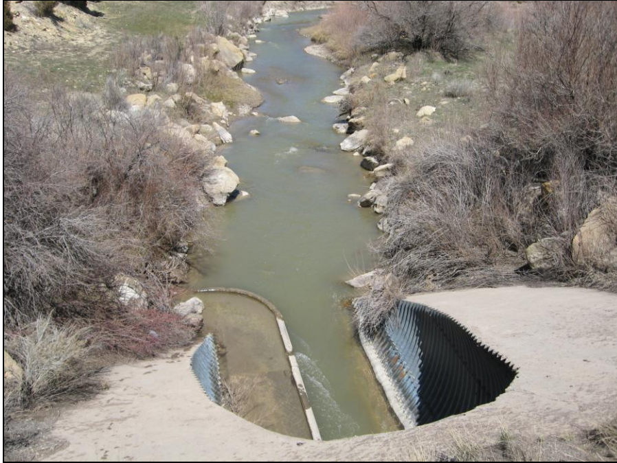
Figure 5-1: Embankment Looking Upstream Photo
