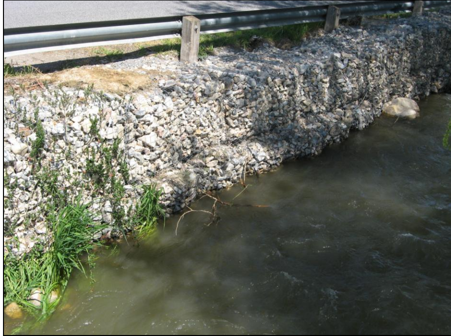
Figure 5-24: Gabion Wall
