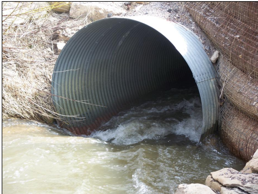
Figure 5-43: Hydraulic Jump Just Inside Culvert Inlet
