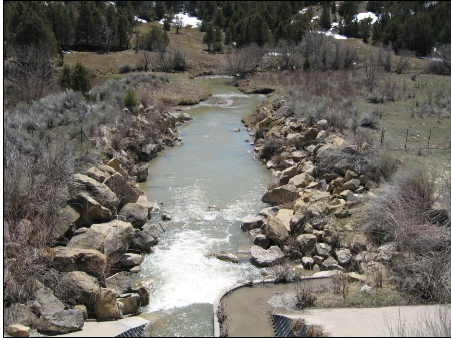
Figure 5-4: Additional Embankment Looking Downstream Photo Showing Floodplain
