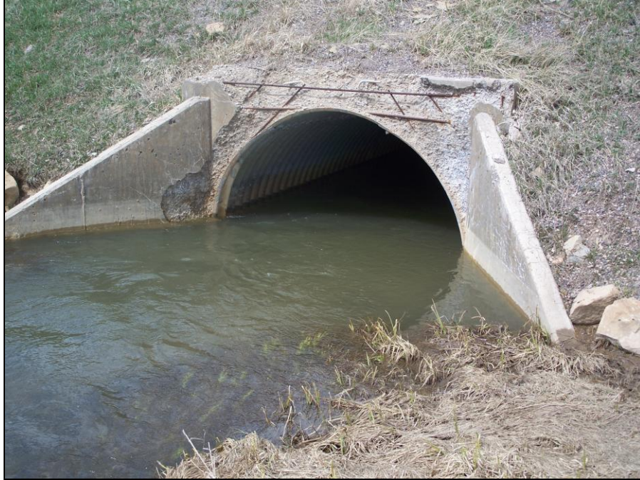
Figure 4-8: Inlet of Backwatered Culvert #1
