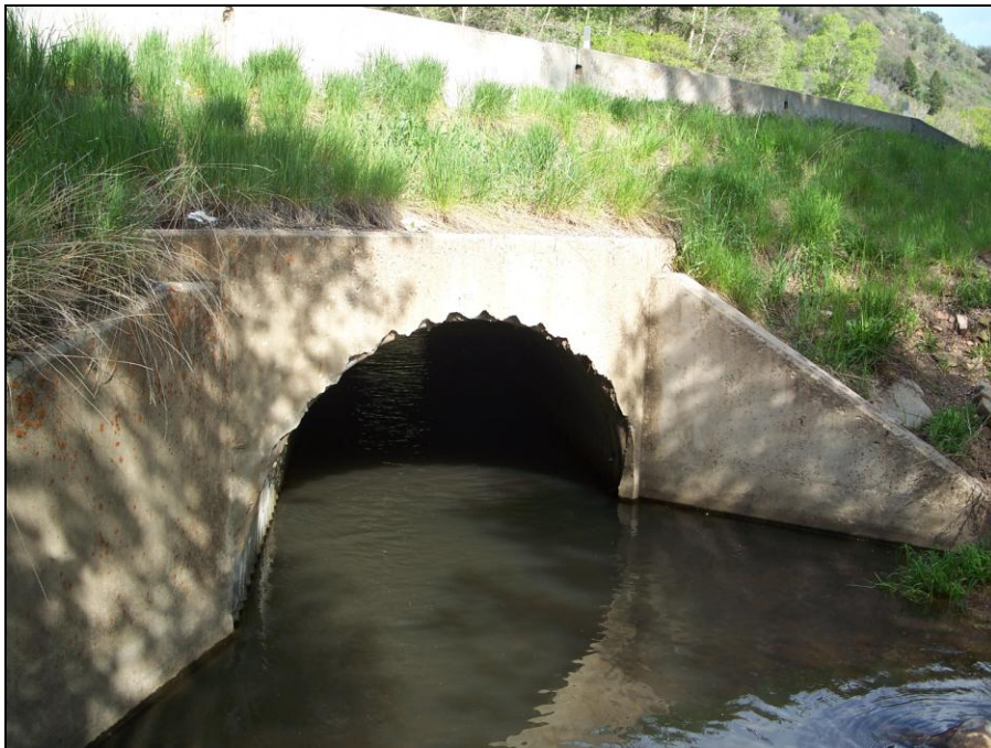
Figure 6-11: Daniel's Creek Culvert #1 Outlet (Daniels Creek Field Verification Site)
