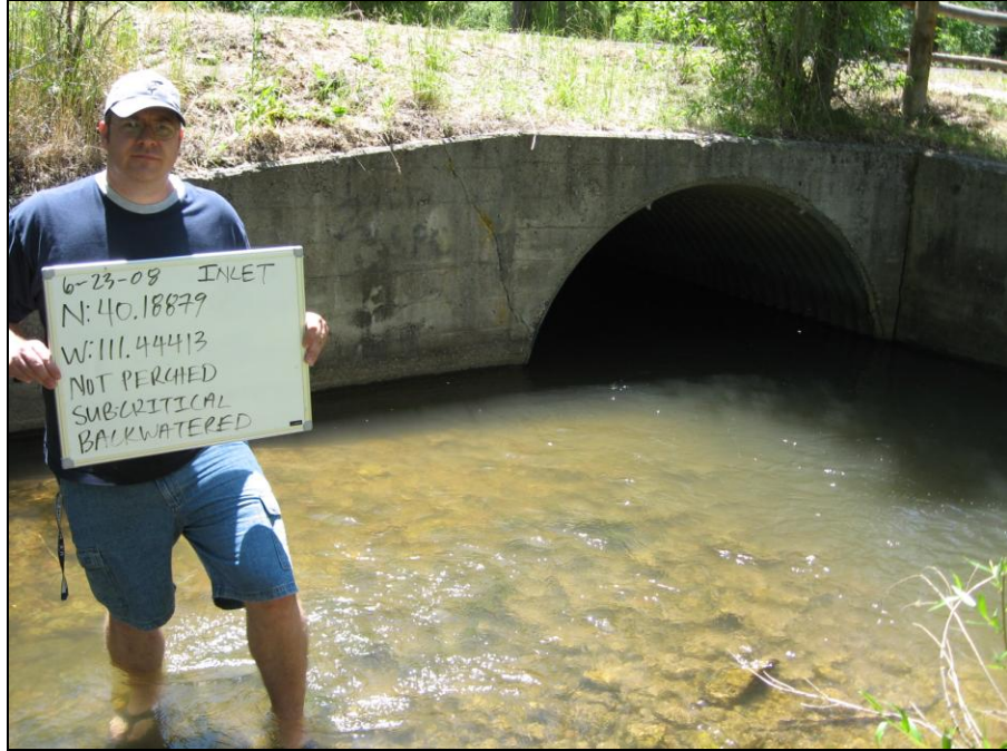
Figure 4-1: Hydraulic Evaluation Photo Taken at the Inlet
