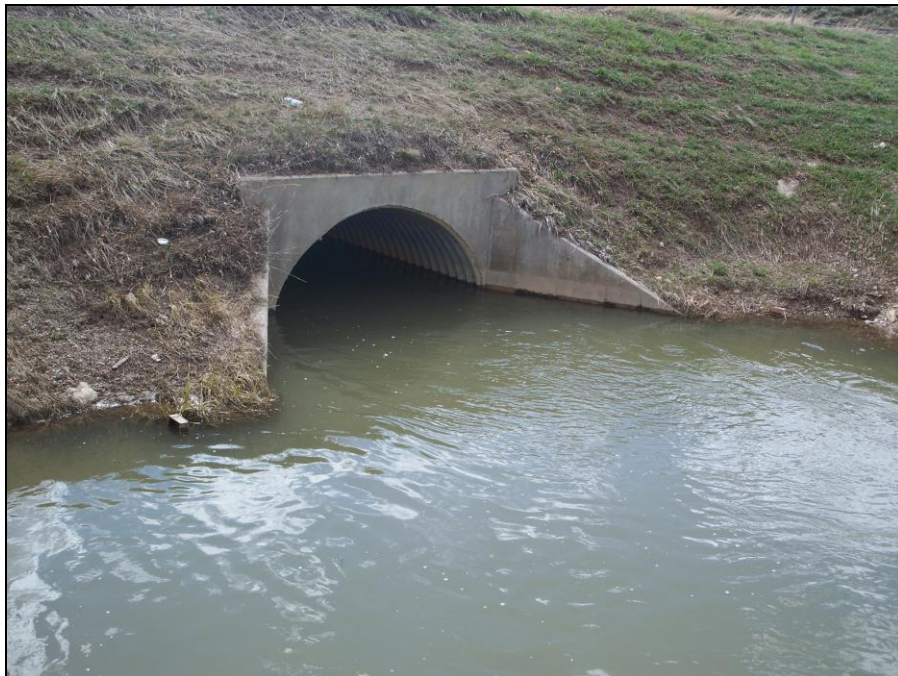
Figure 4-9: Outlet of Backwatered Culvert #1
