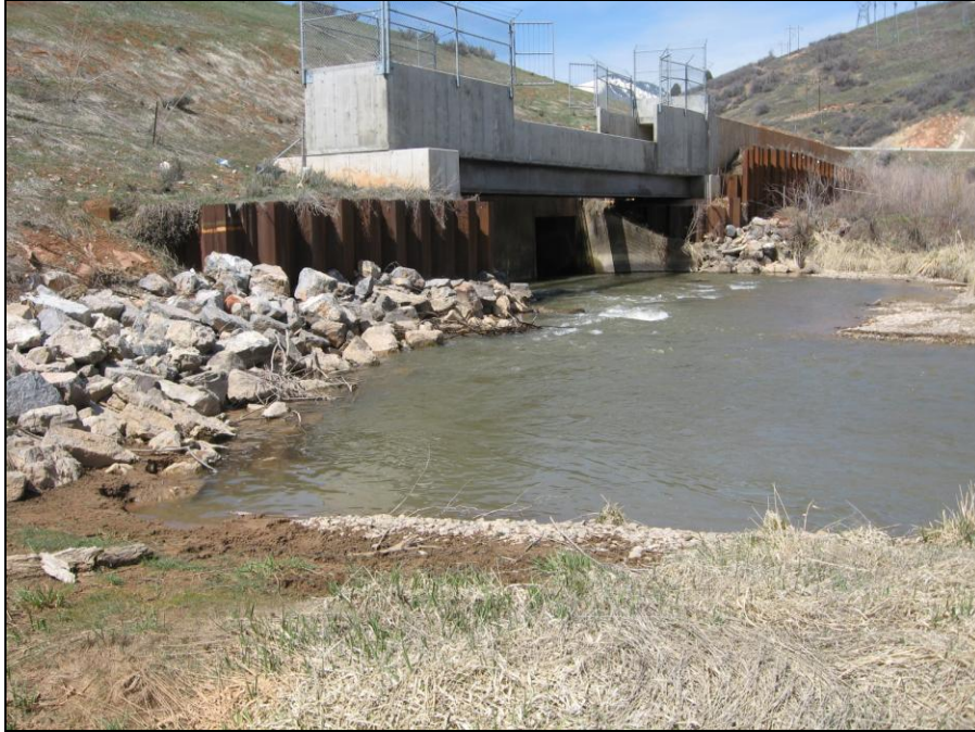
Figure 5-22: Riprap and Sheet Pile Near Inlet
