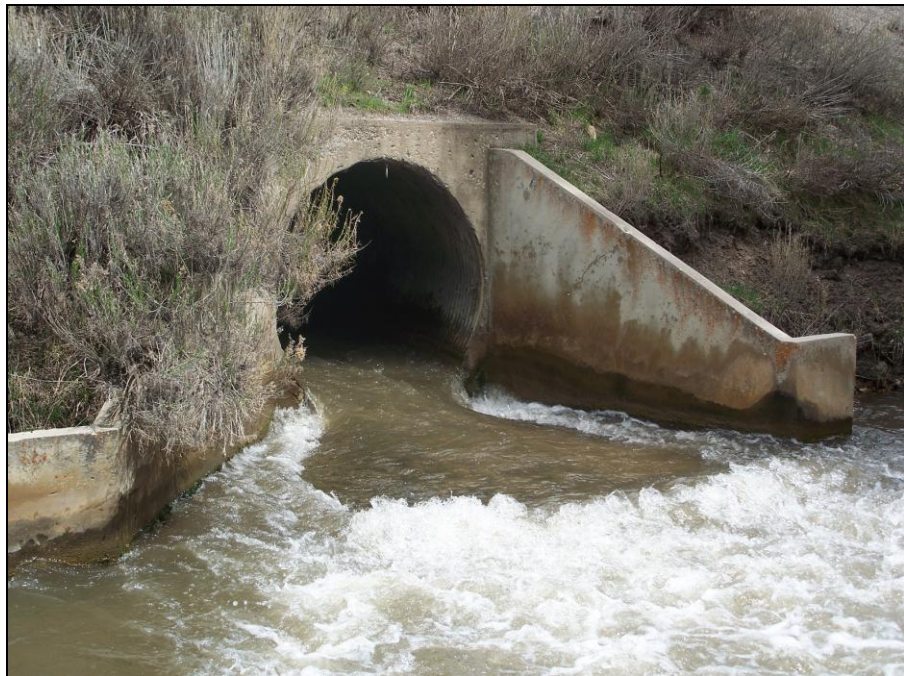
Figure 5-45: Hydraulic Jump at End of Outlet Apron
