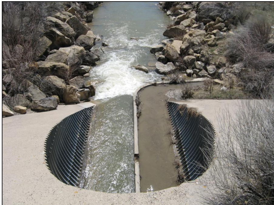
Figure 5-3: Embankment Looking Downstream Photo
