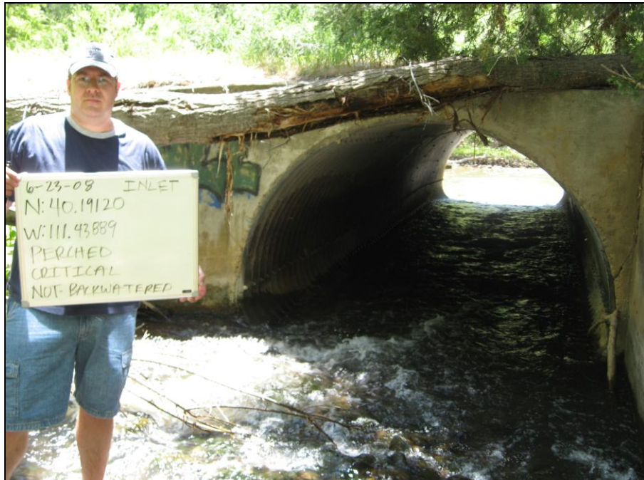
Figure 3-6: Hydraulic Evaluation Photo of a Culvert Inlet
