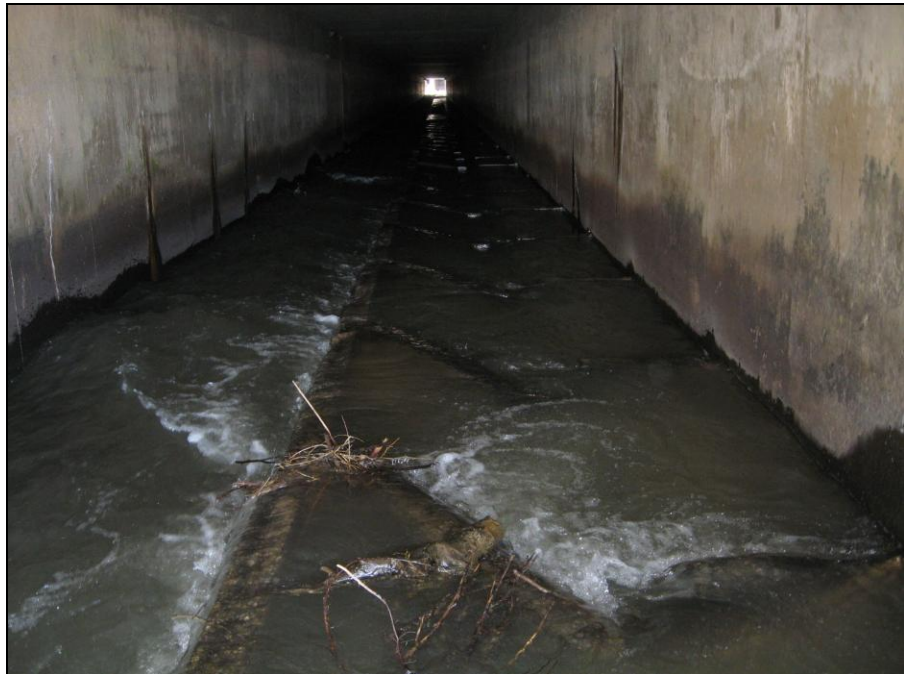
Figure 5-12: Photo of Fish Baffles Mid-Culvert
