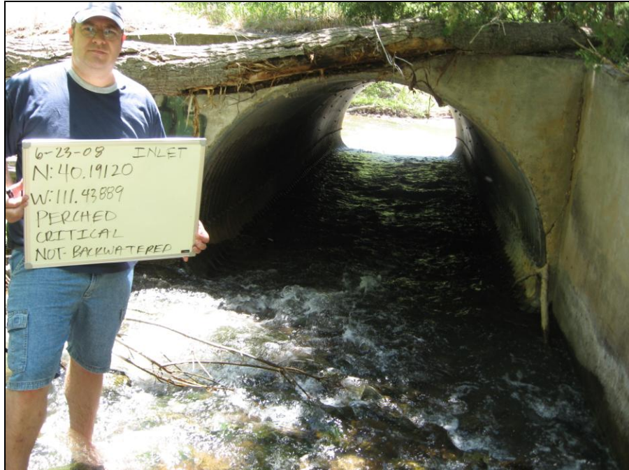
Figure 4-3: Hydraulic Evaluation Photo Taken at the Inlet
