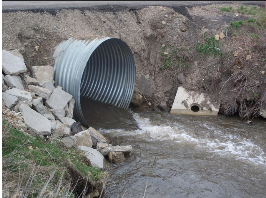
Figure 5-44: Hydraulic Jump Just Downstream of Outlet
