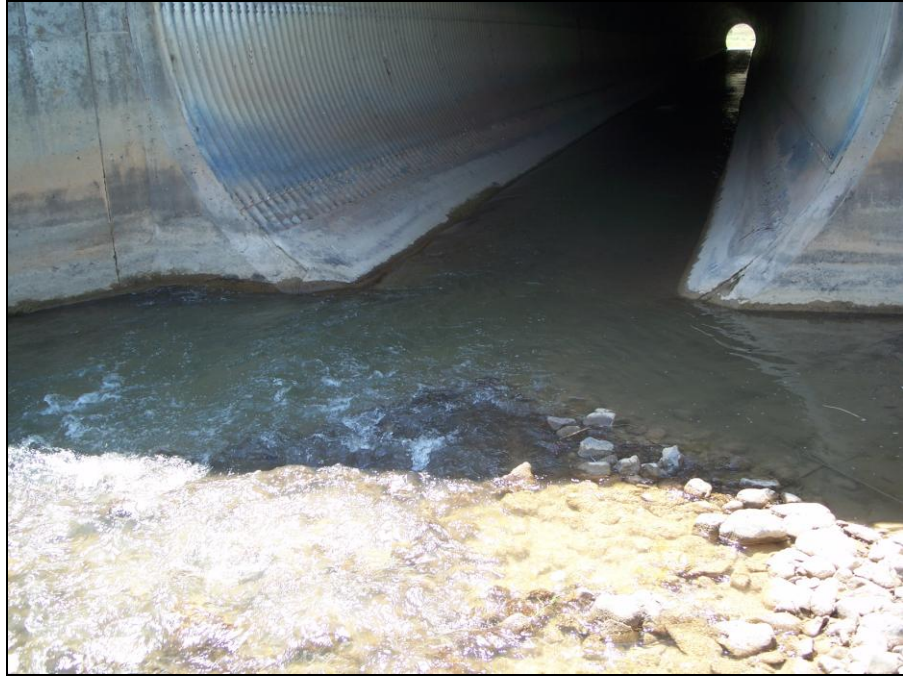
Figure 4-10: Inlet of Backwatered Culvert #2
