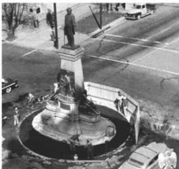
Reducing the base of the monument in 1956. The stone eagle and beehive at the lower right are decorations at the top of one of four lightposts installed in 1947. Located on the intersection's corners, these were specially placed to light the monument.
