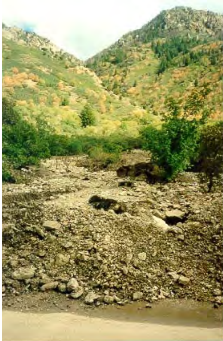
Figure 8: The September 8 Preston Canyon debris flow where it crossed Preston Canyon Drive; Preston Canyon is visible in the background. Photograph taken facing east. (September 18, 2002)
