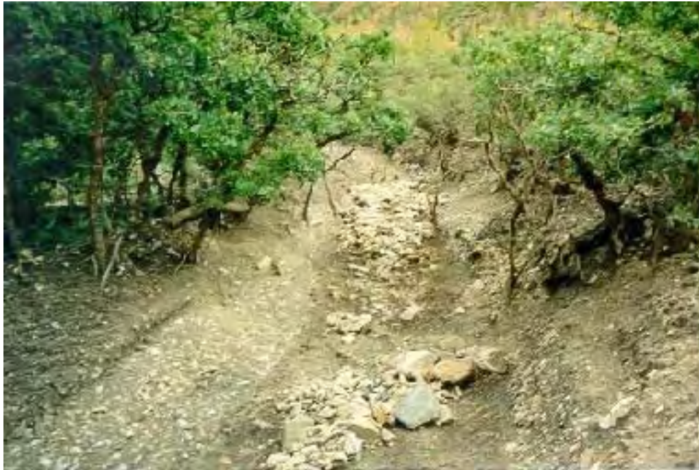
Figure 12: The channel of the Preston Canyon debris flow, photograph taken facing east. (September 18, 2002)
