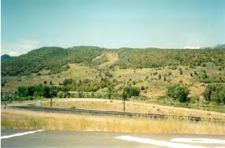
Figure 18: Shurtz landslide, photograph taken facing west. Only the two earthflows are visible, the remainder of the slide is on the plateau. (July 4, 2002)
