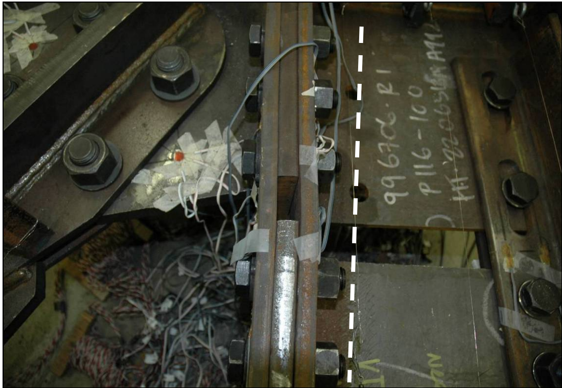
Figure 3-6 Specimen 1 – Splice Plate Deformation Following Boundary Failure
