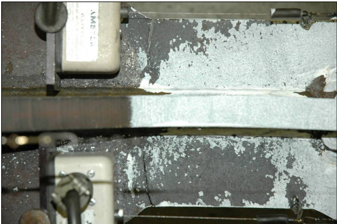
Figure 3-27 Specimen 2 – BRB Core Extension Fracture (6.5% Drift Fatigue Cycles)
