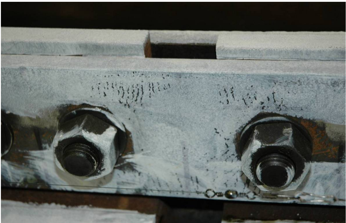
Figure 3-19 Specimen 2 – Initial Yielding of Splice Plate (2% Drift)
