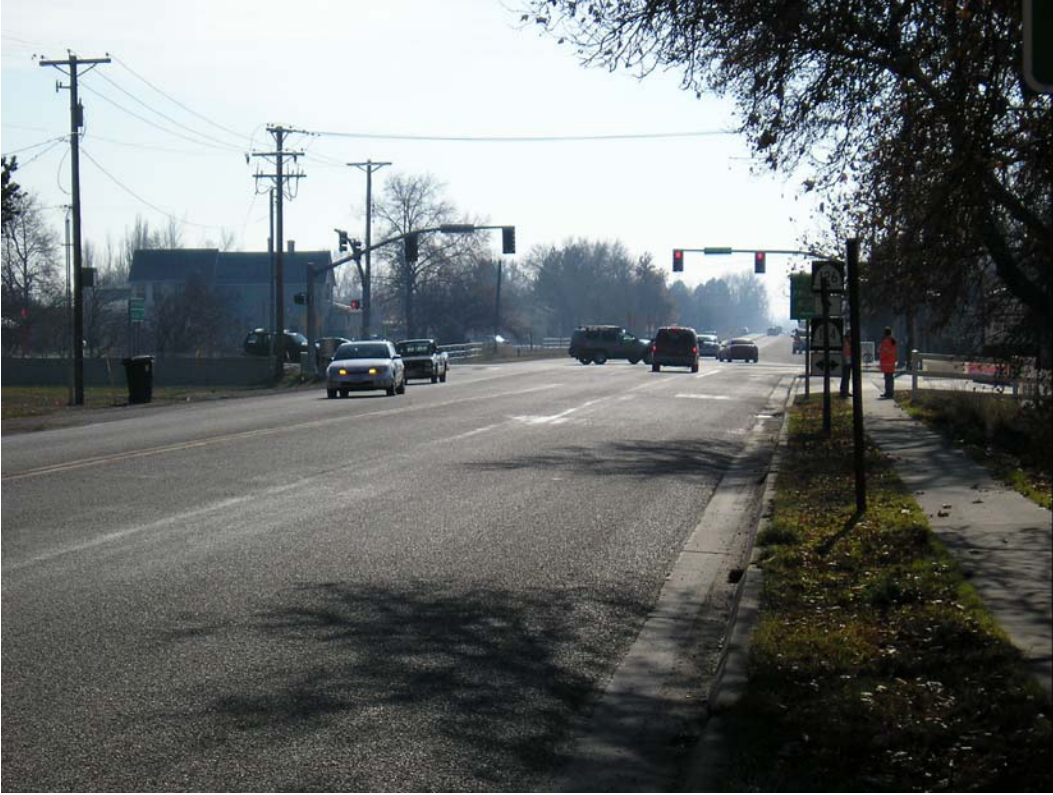
Figure 4.7 Intersection of S.R. 126 & S.R. 134 in Farr West.
