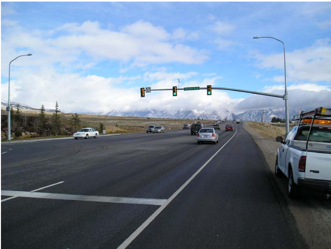
Figure 4.13 Intersection of S.R. 92 & Triumph Boulevard in Lehi.
