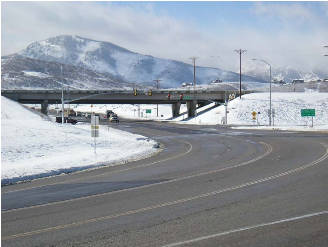
Figure 4.9 Intersection of S.R. 248 & S.R. 40 near Park City.
