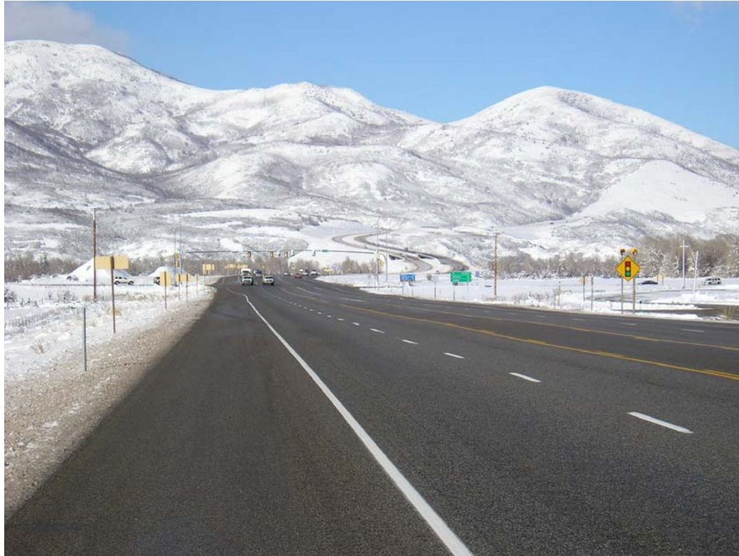
Figure 4.16 Intersection of S.R. 40 & S.R. 32 in Heber.
