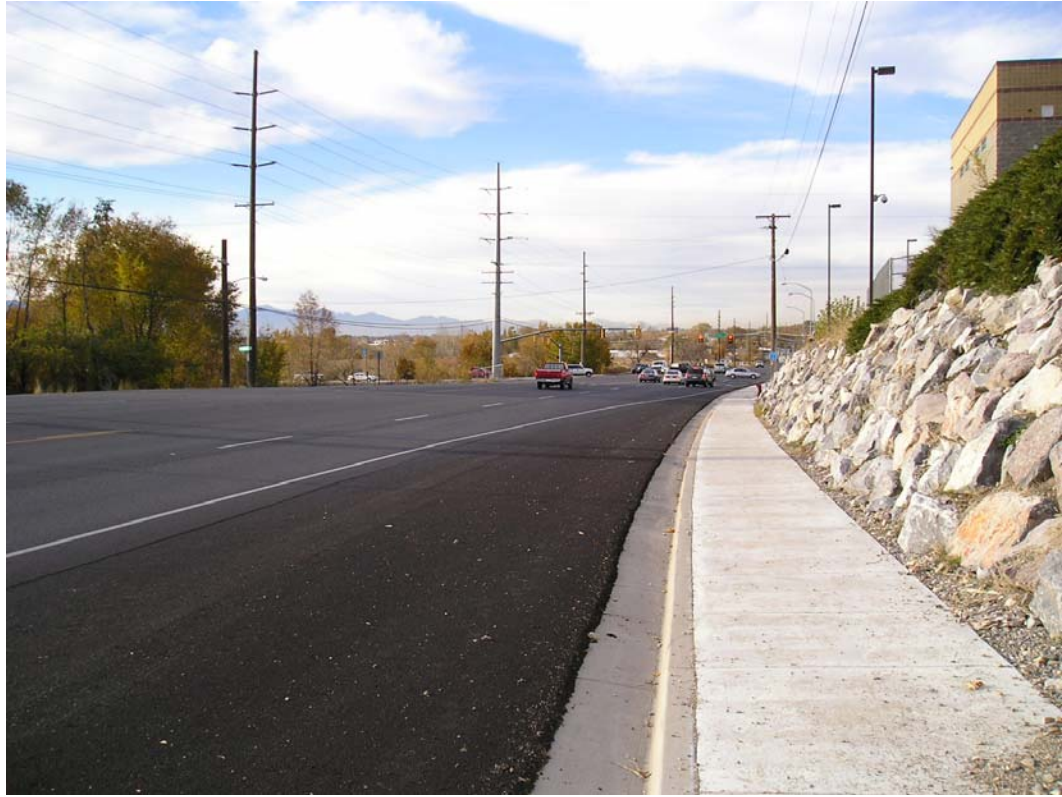
Figure 4.18 Intersection of S.R. 89 & 1860 South in Provo.
